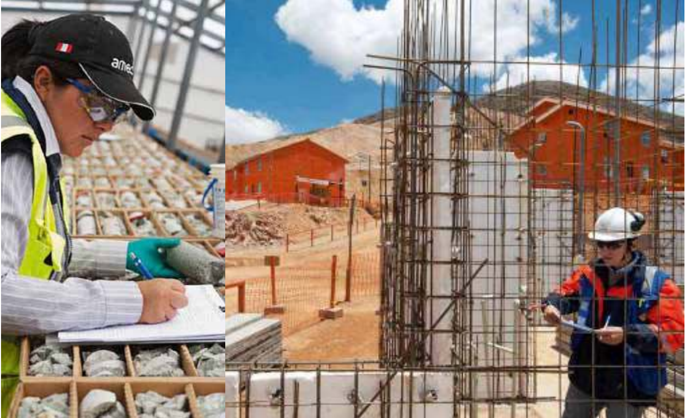
Left: Samples are analysed as part of the Coroccohuayco project. Right: Contractor works on construction of Nueva Fuerabamba.
