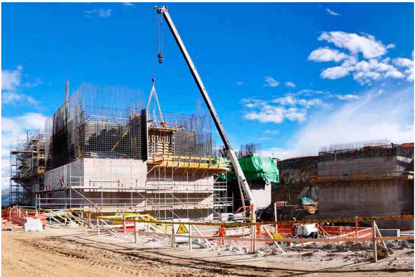
Construction of the concentrator plant at Las Bambas.
