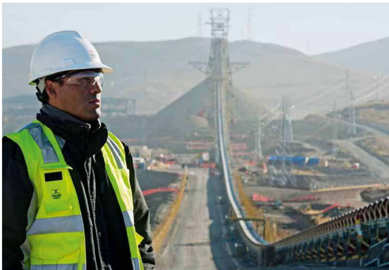
Ore is carried by conveyor belt to the concentrator plant at Antapaccay.
