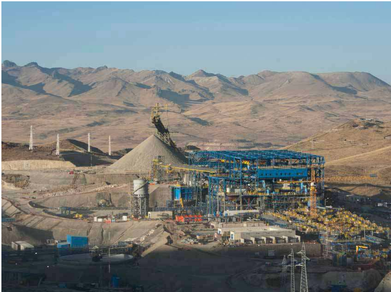
Modern concentrator plant at Antapaccay.
