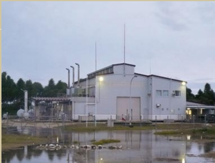
Tuvalu Electric Power (TEC) Building, Funafuti, Tuvalu.
