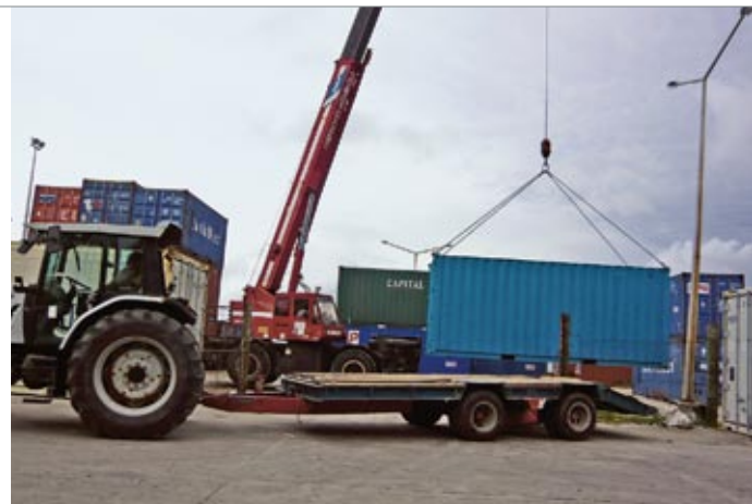
Construction material container transportation at the Funafuti harbour.
