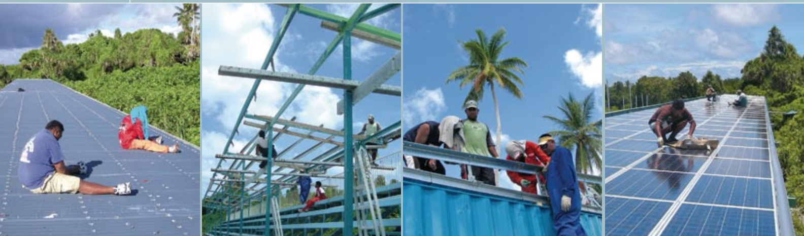
Project implementation and construction phases.
