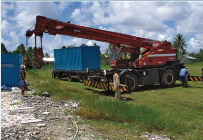
Construction material transportation on site.
