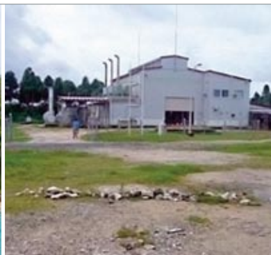
Tuvalu Electric Power (TEC) Building, Funafuti, at low tide.
