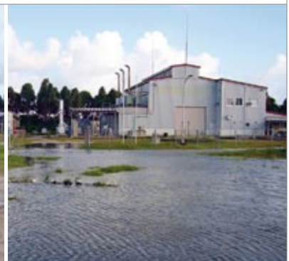
Tuvalu Electric Power (TEC) Building, Funafuti, at high tide.
