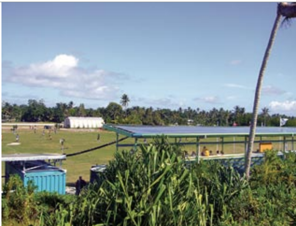
The e 8 Tuvalu Solar Power Project site.
