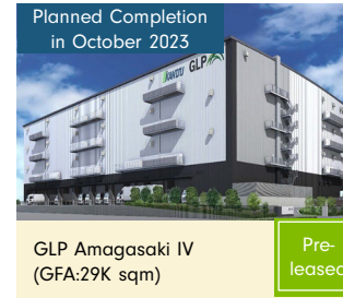
Planned Completion in October 2023 GLP Amagasaki IV (GFA:29K sqm)
