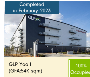
Completed in February 2023 GLP Yao I (GFA:54K sqm)
