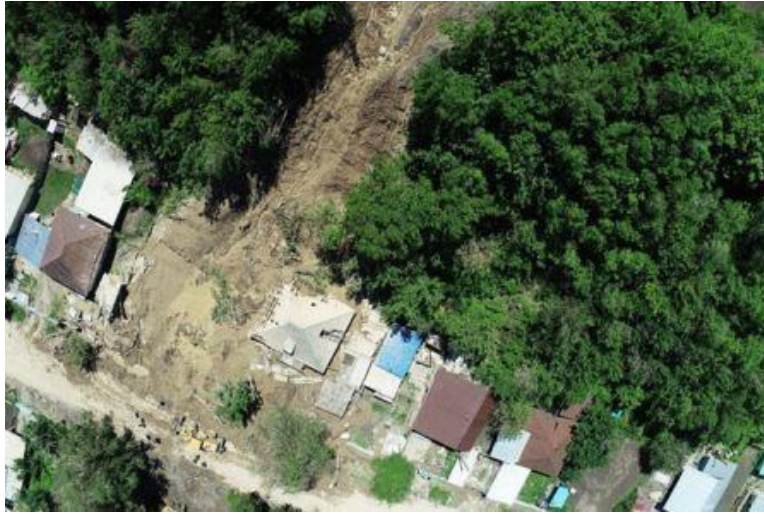
Fig. 8: Landslide deposition zone
