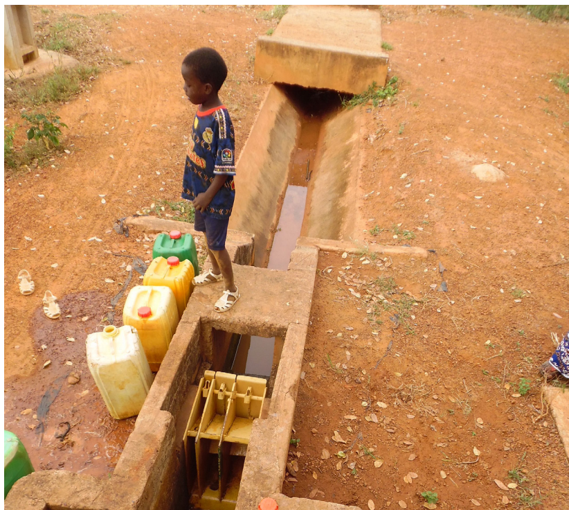
Baffle distributor, Bafoulabé, Kayes, Mali.
