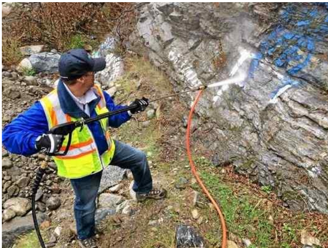
Figure 3. Graffiti cleanup in the canyon
