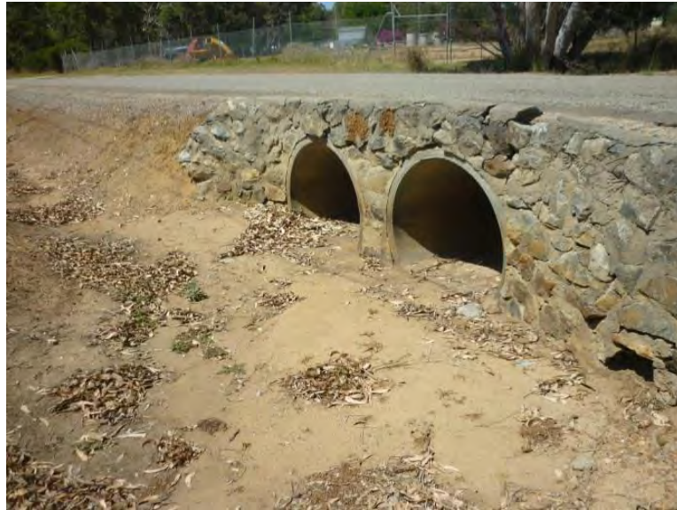
Plate 6 Culvert beneath Grove Road
