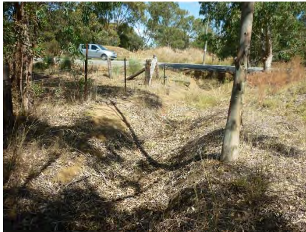
Plate 3 Existing drainage channel
