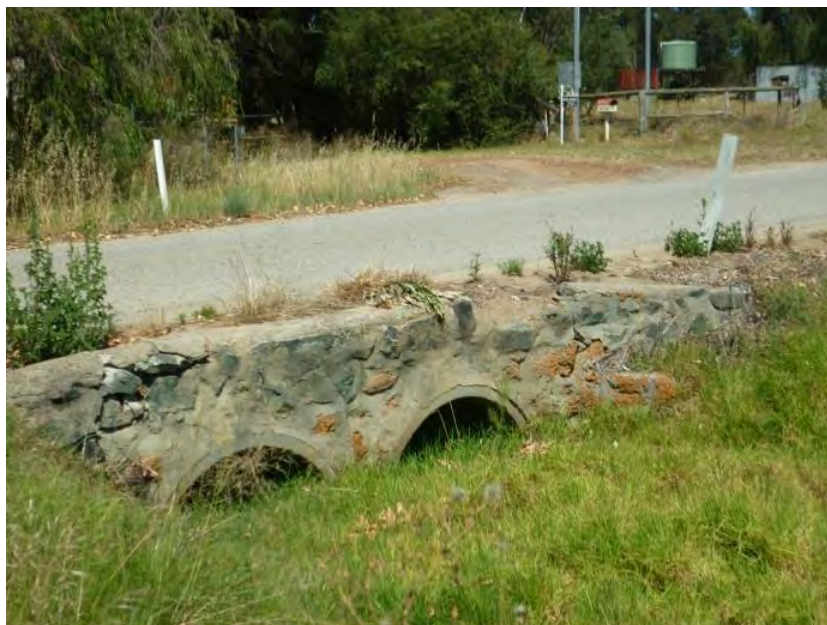
Plate 5 Culvert beneath Edward Street
