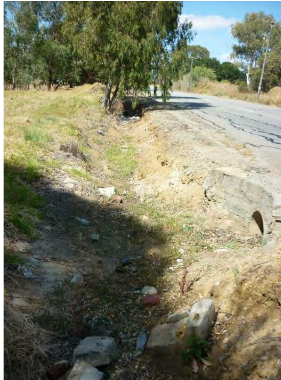
Plate 2 Road verge swale
