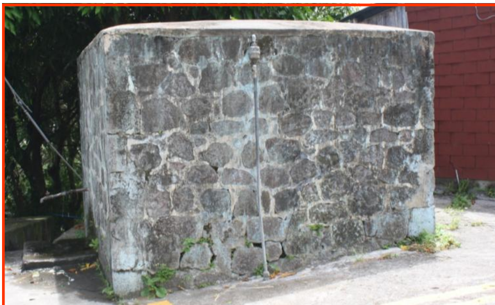
St. John's Water Tank
