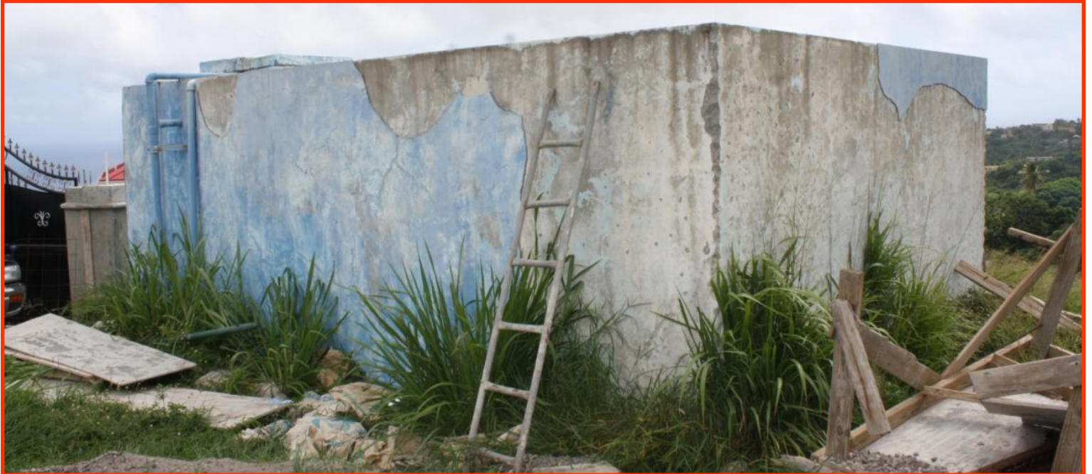
Baker Hill Water Tank
