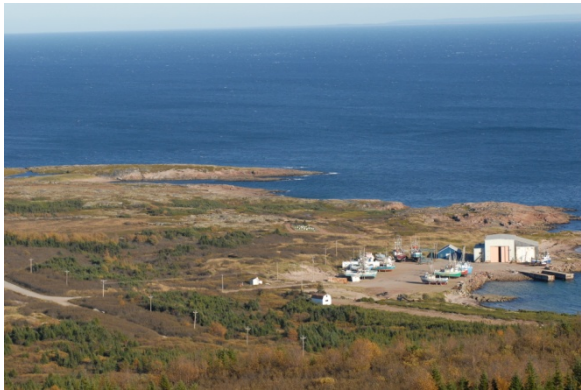
Aerial image of the L'Anse au Diable electrode site
