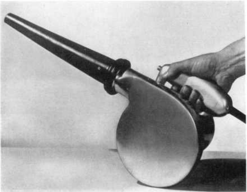
FIGURE 8.—Blower for use in cleaning seed dividers.
