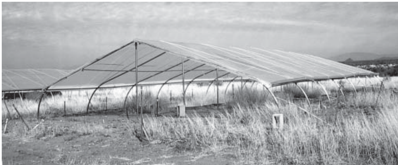
Figure 1 —Shelter (9 by 18 m, 4 m tall) on the Pleistocene site; open sides are 1.5 m off the ground. Tall grasses visible beneath the shelter are Heteropogon contortus . Note the cables attached to the shelter and steel fenceposts for greater wind stability, and polypropylene rope holding down the plastic cover.
