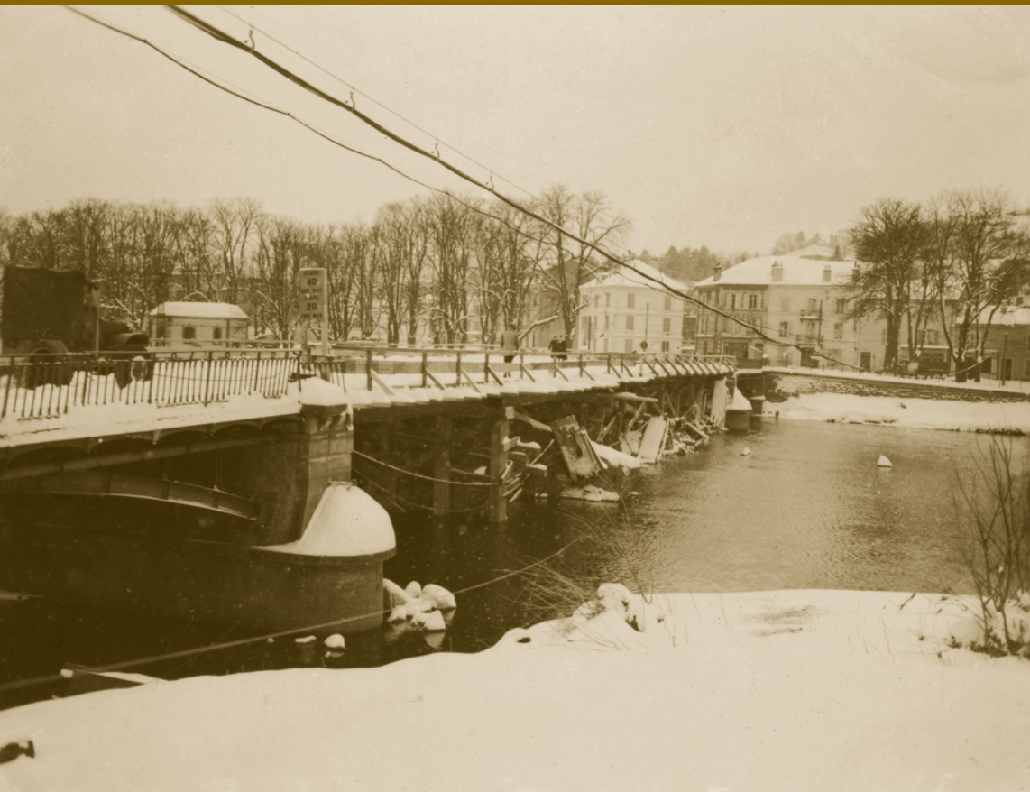
Bridge over the Moselle River, rebuilt by Company B of the 1321st in Epinal, France, 27 January 1945.
