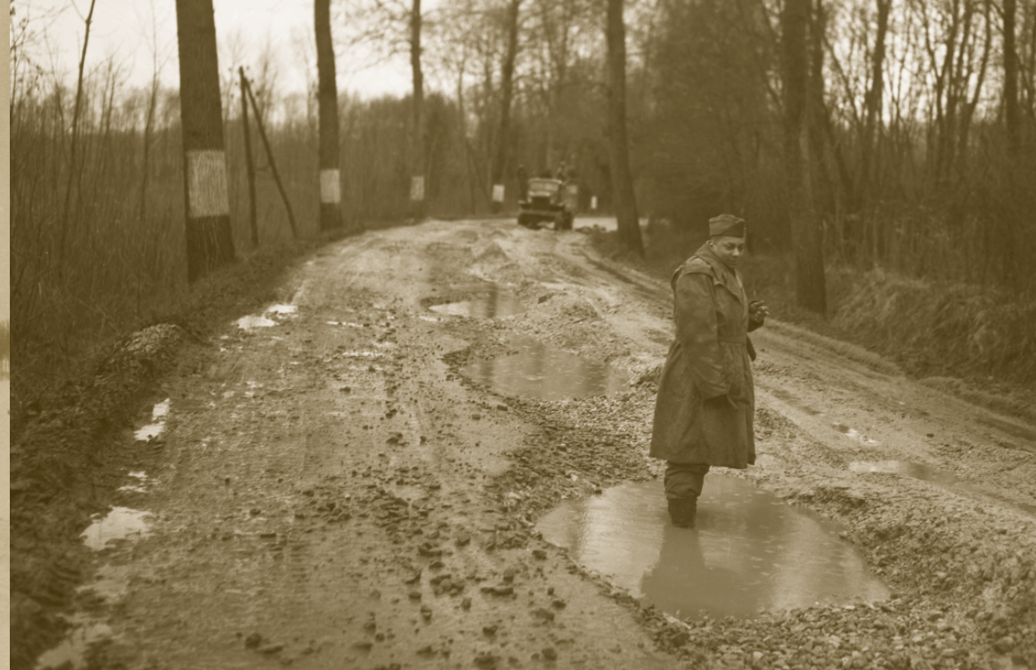
Shin deep in rain and mud, an engineer inspects road damage from spring thawing and heavy vehicle use.
