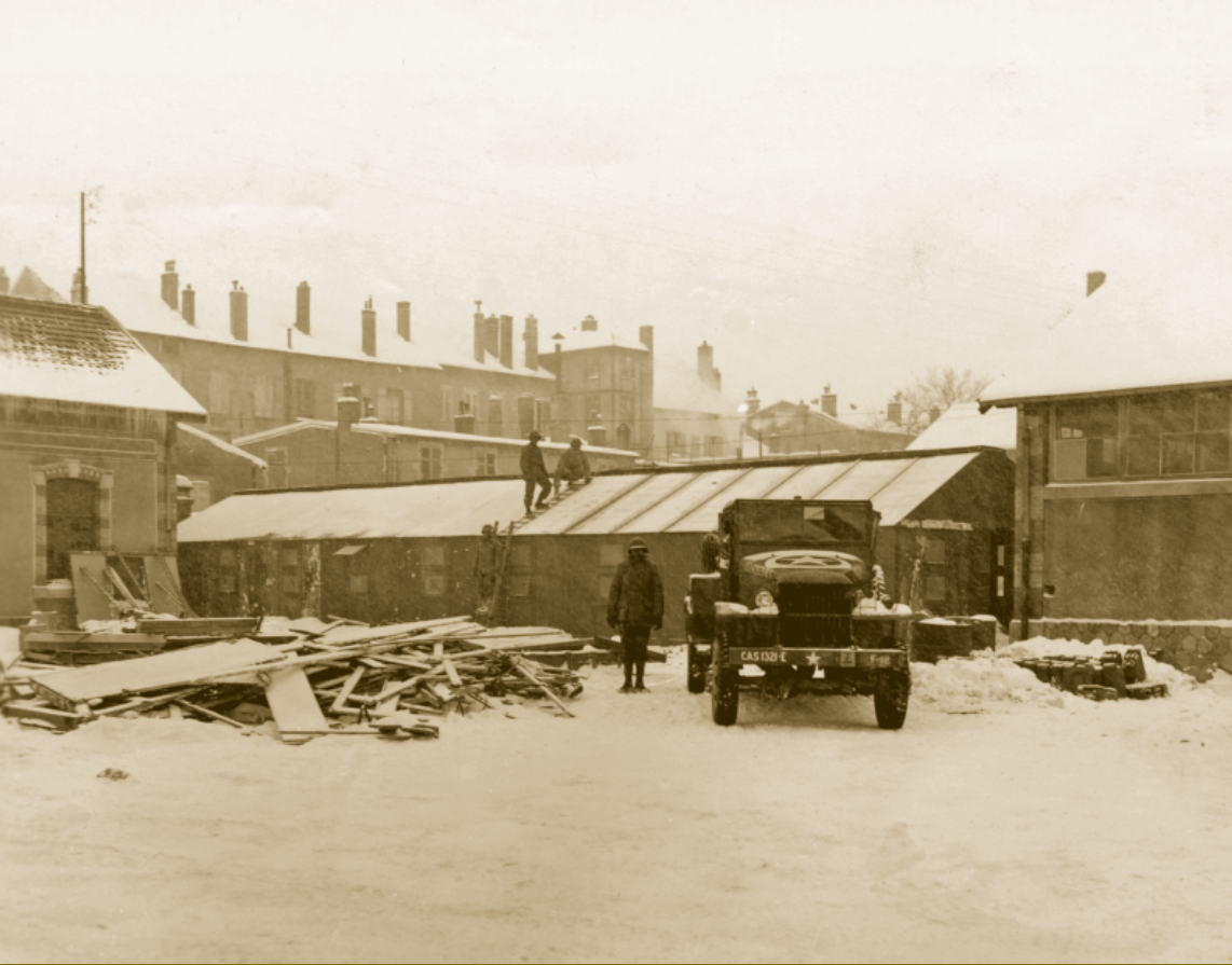
Hospital construction using prefabricated components in Lunéville, France, 30 January 1945.
