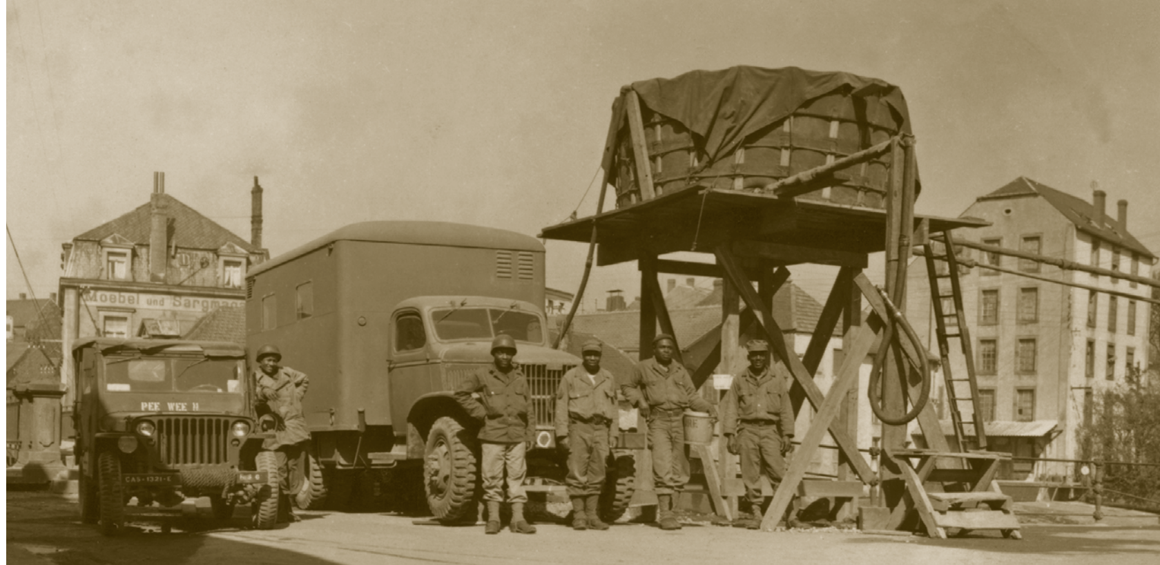
Engineers of the 1321st and a newly completed water point, which purified and distributed potable water, 8 April 1945.
