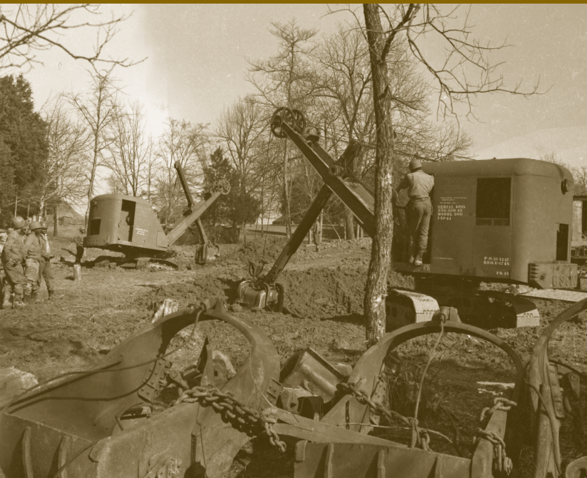
Soldiers training on dragline power shovels, used primarily by the 1321st for quarrying and excavation.
