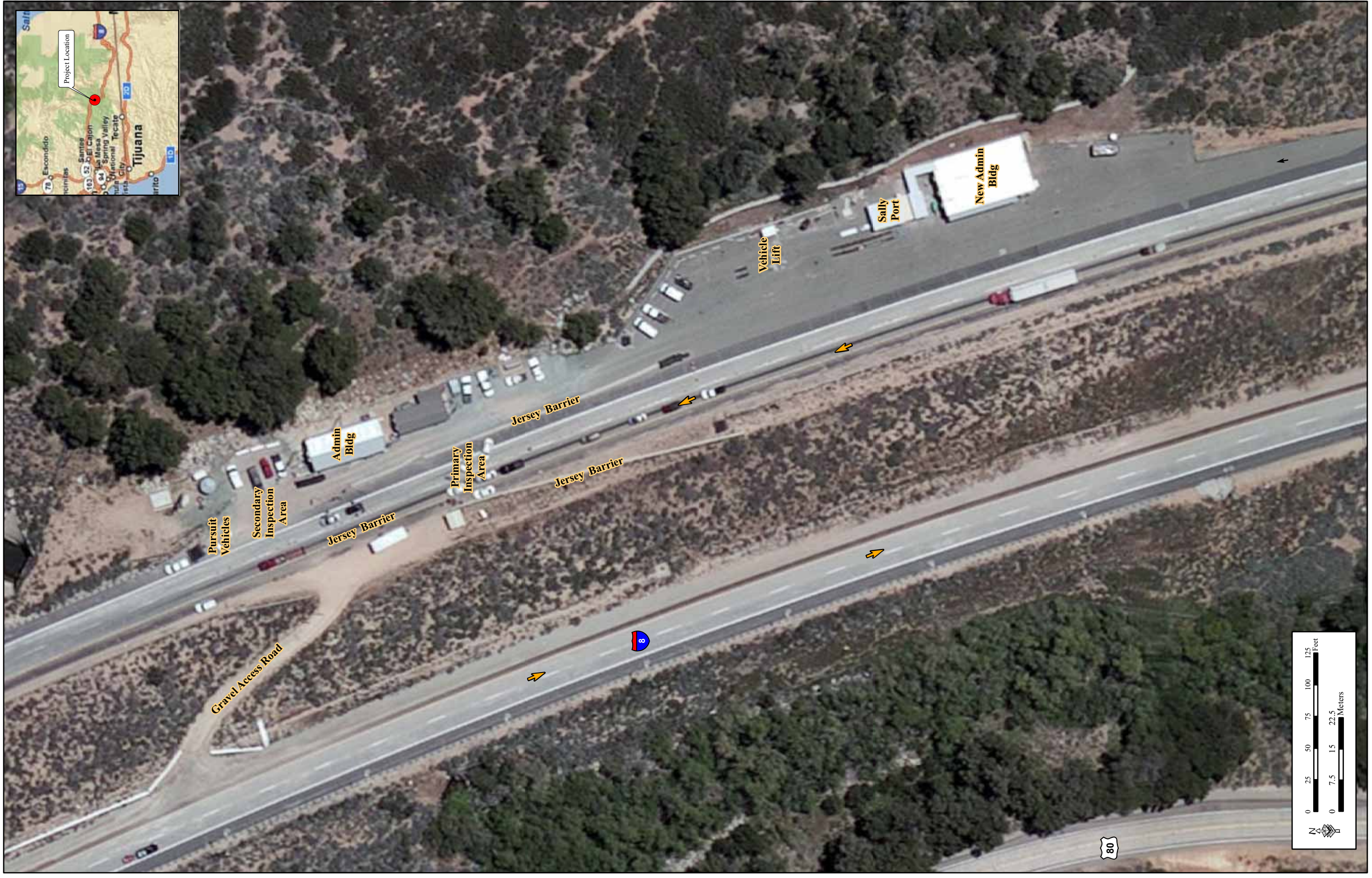
Figure 2-1. Existing Facilities at I-8 Checkpoint
