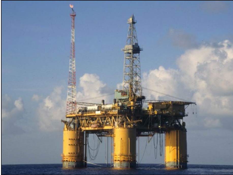
Figure 3.31. Conoco's Jolliet tension-leg well platform (or TLWP), set in 1,722 feet of water, began oil and gas production in 1989.
