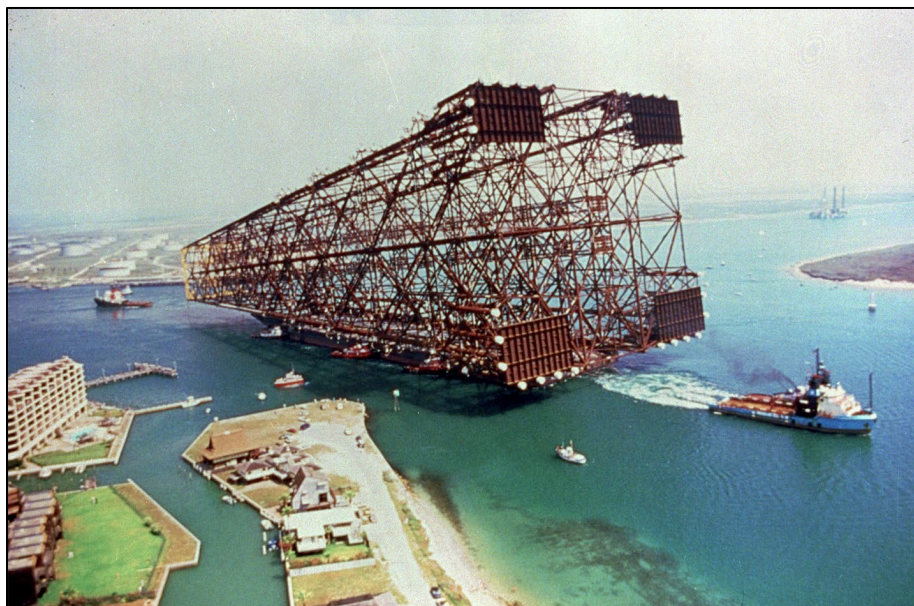
Figure 3.29. Shell Oil's monumental Bullwinkle production platform dwarfs a Corpus Christi hotel being transported in January 1987 from Texas to its target site in the deepwater Gulf.
