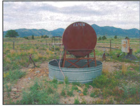
Figure 15: Above ground storage tank.
