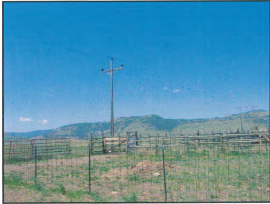
Figure 4: Electric transmission lines along the southern property boundary.
