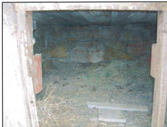
Figure 8: Interior of bunker.
