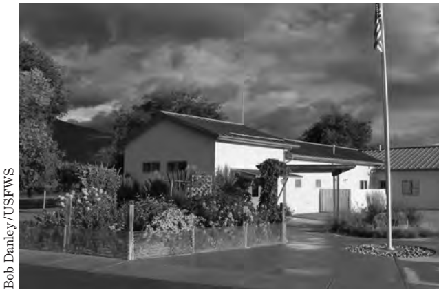
The refuge's existing headquarters would be expanded to include additional office space and a combined classroom and conference room.
