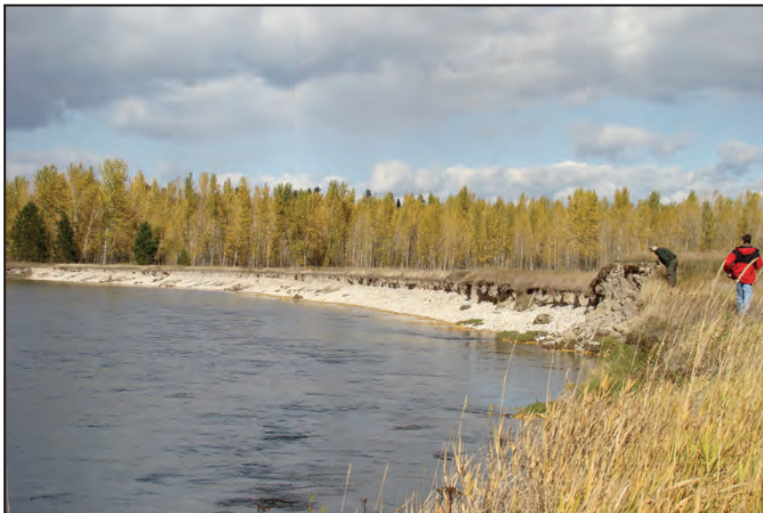
Figure 16. Bank and levee erosion along the Bitterroot River on the west side of Lee Metcalf National Wildlife Refuge, Montana (Heitmeyer et al. 2010).
