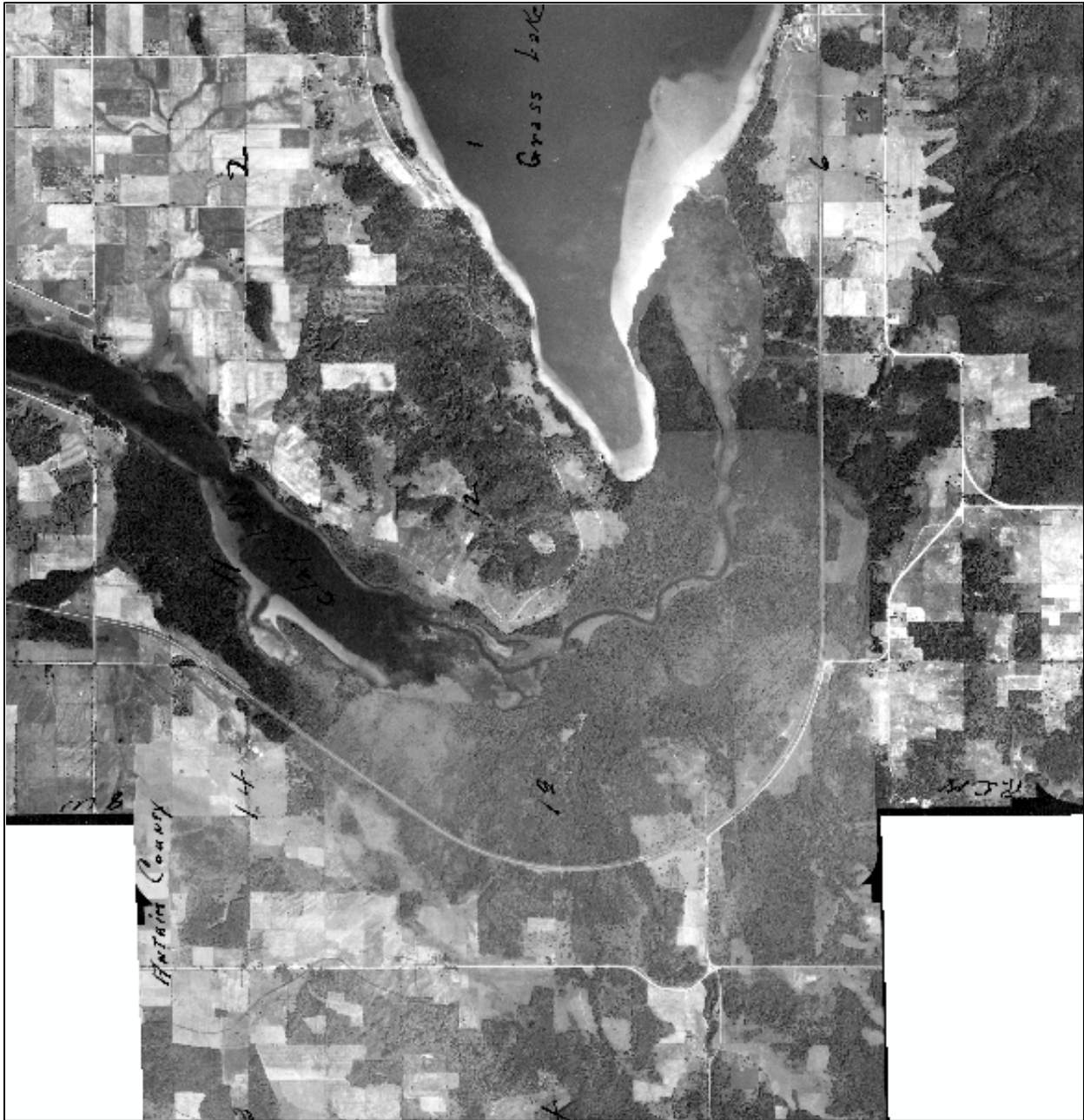
Figure 48. 1938 aerial imagery showing extensive cutting of both upland and lowland forests in GRNA and the surrounding environment.
