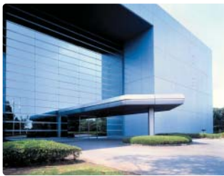
CTC data center
