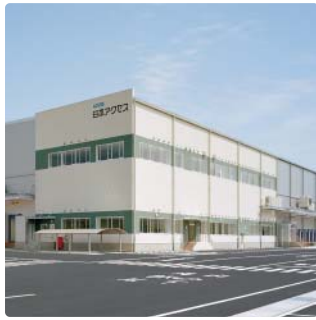
NIPPON ACCESS, INC.'s Hiroshima Low Temperature Center
