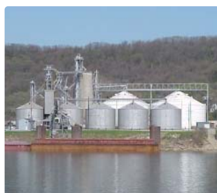
River grain elevator of CGB Enterprises, Inc.
