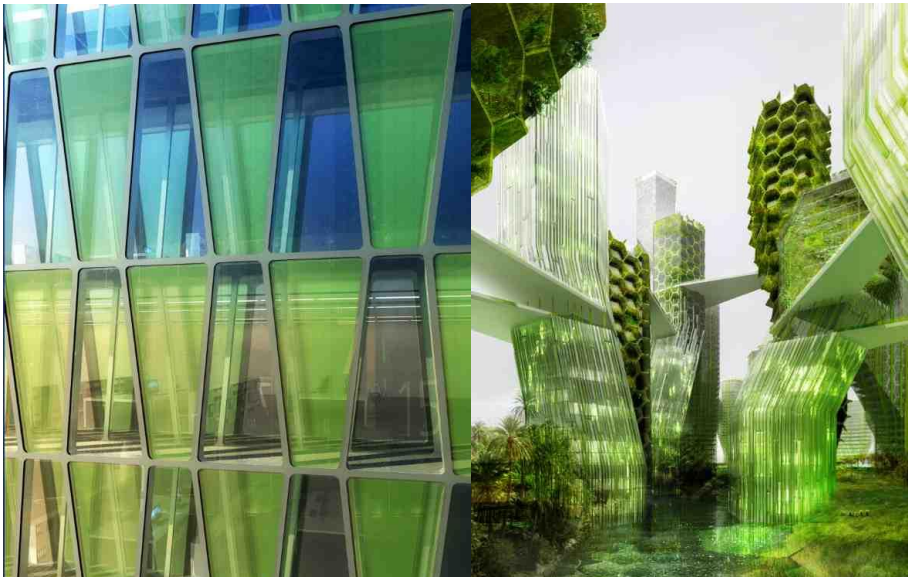
Fig. 3 – Biofaçade (left), detail, photo-bioreactors integrated architecturally and technically in the curtain wall, 2011, © XTU Architects. X Sea Ty Centre (right), concept for a sustainable city, 2009, © XTU Architects, www.x-tu.com
