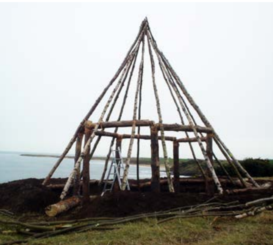
Illustration 4.4a: Reconstruction in progress at Howick © Clive Waddington
