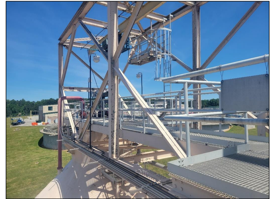
End of bridge truss, crane elements and walkway #1
