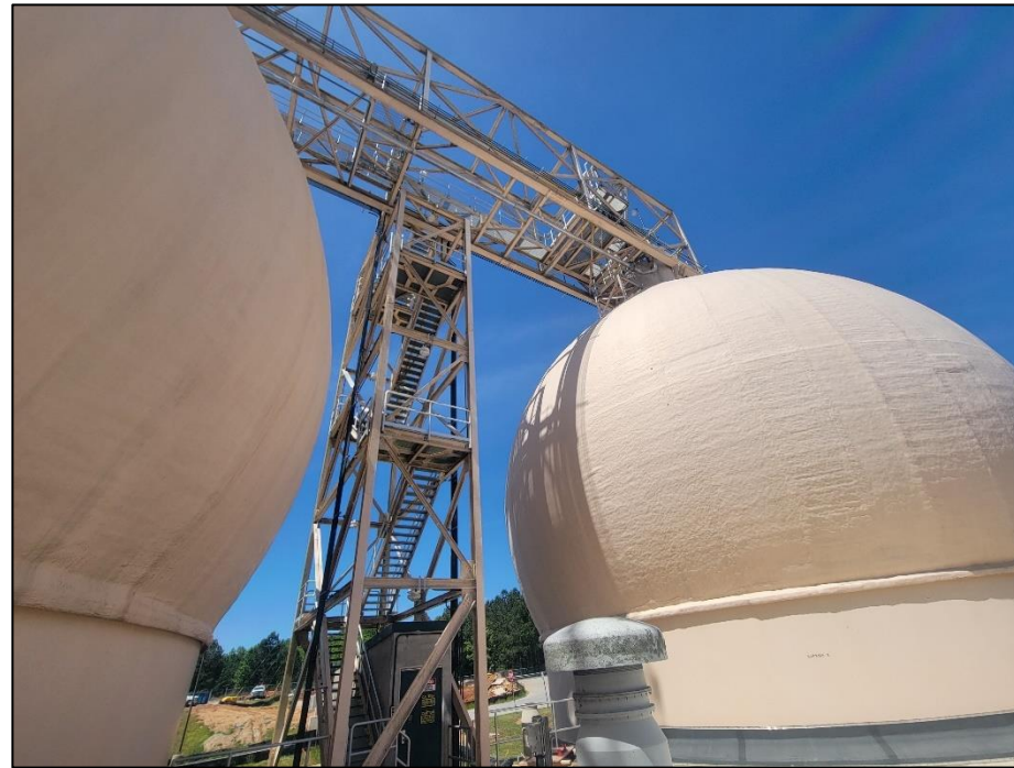
Stair tower at bridge truss walkway #1
