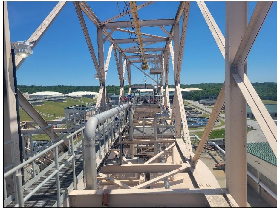
Bridge truss, crane elements and walkway #4
