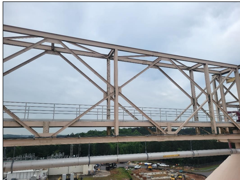
Bridge truss and walkway #2
