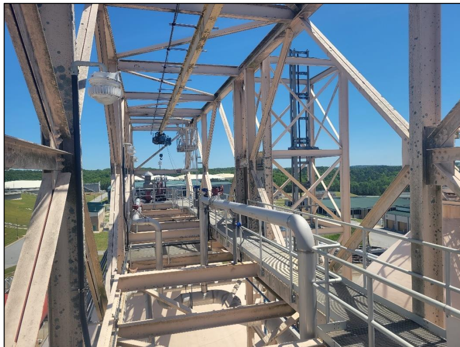
Bridge truss, crane elements and walkway #3
