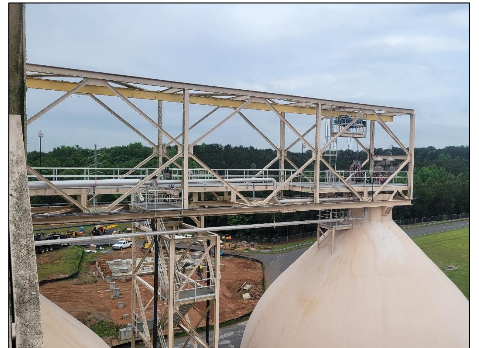
Bridge truss, crane elements and walkway #1
