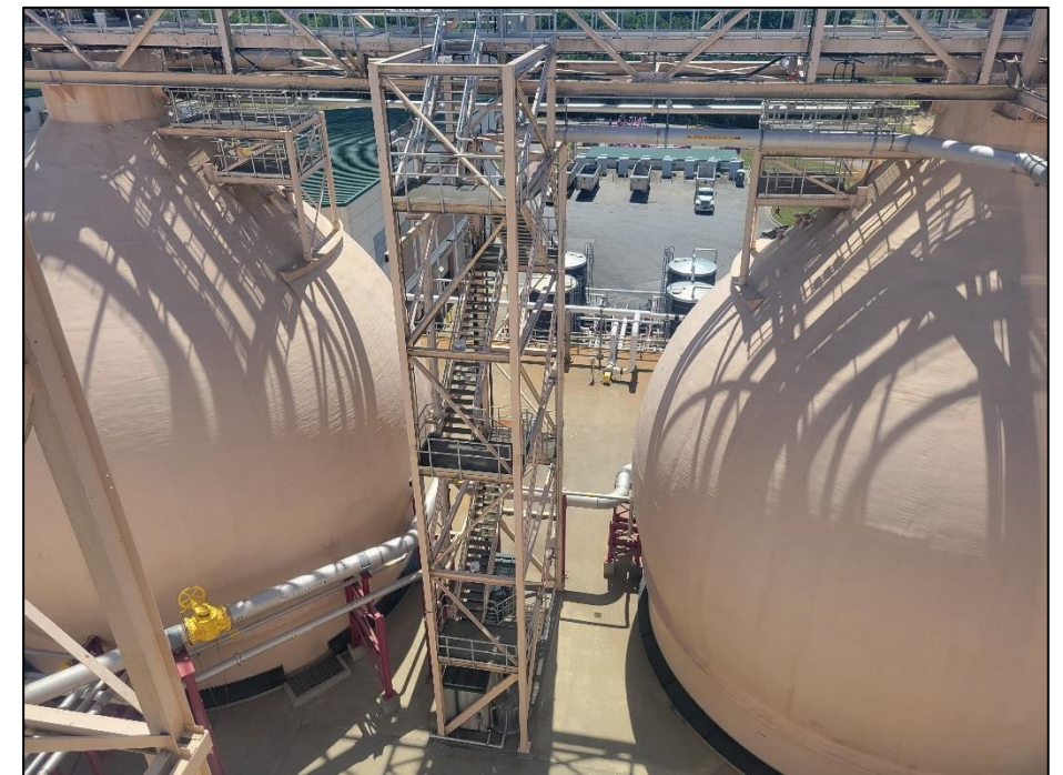
Stair tower at bridge truss and walkway #4
