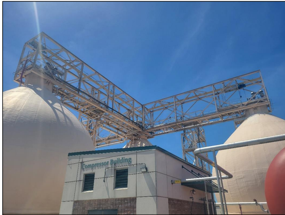
Bridge truss, crane elements and walkways #1 and #3
