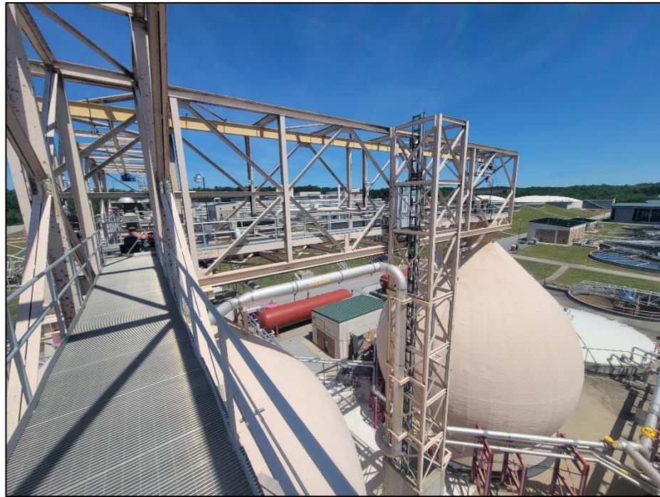
Bridge truss, crane elements and walkway #3
