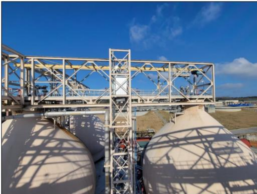
Figure 5: View of elevator tower and truss bridge/walkway between Digesters 4 and 5.
