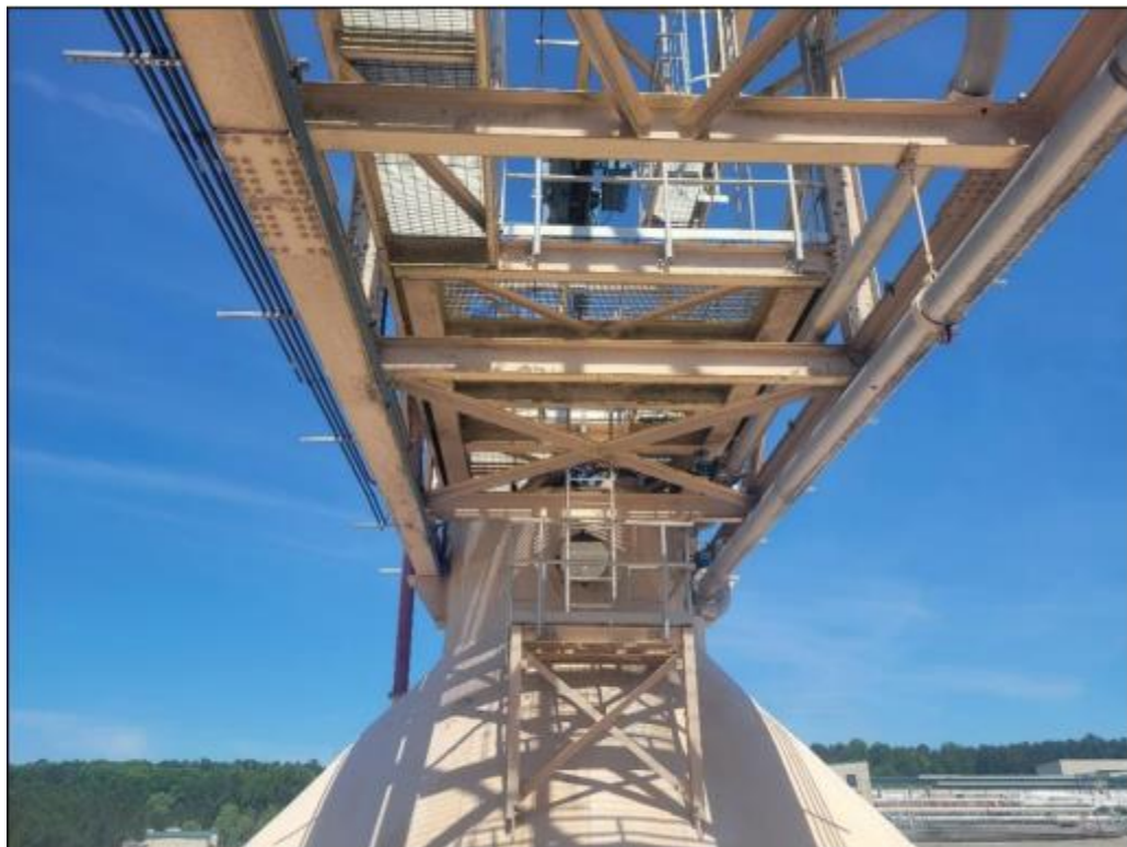
Figure 3: View of bottom chords looking towards Digester #3.
