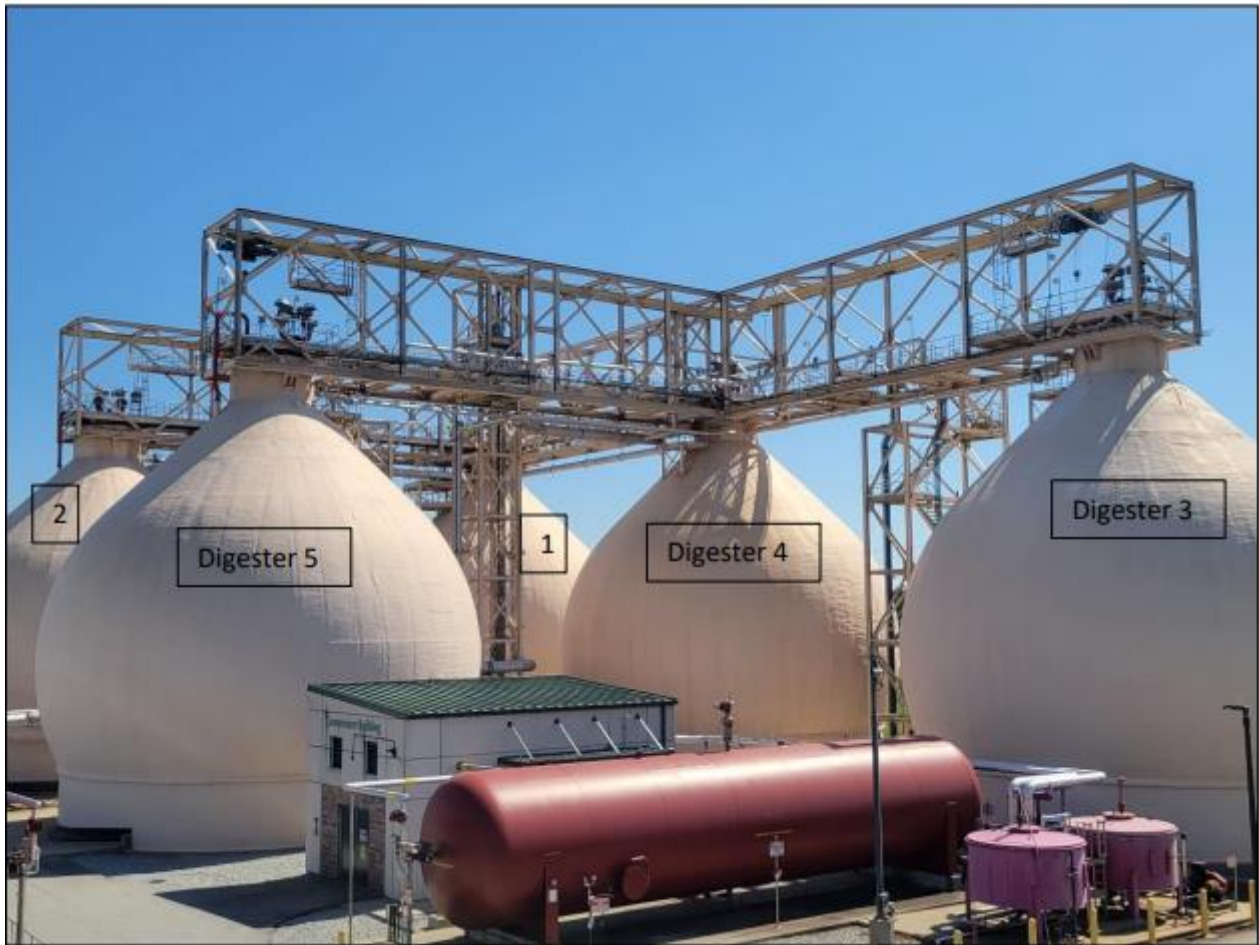
Figure 2: Wide angle view of Digesters and Steel Super Structure
