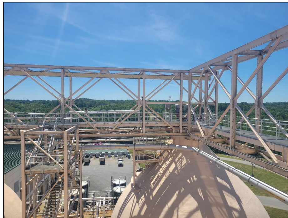
Bridge truss, crane elements and walkways #2 and #4
