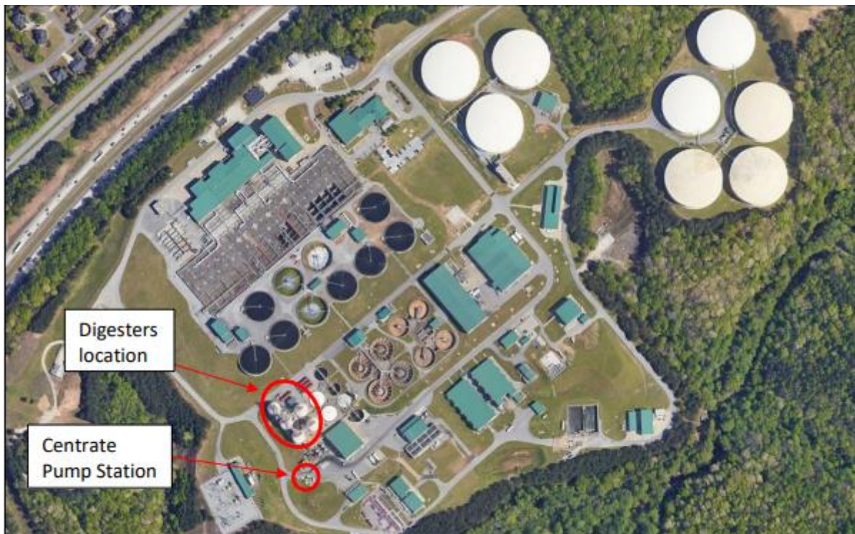
Figure 1 – F. Wayne Hill WRC Digesters Facility & Centrate Pump Station locations
