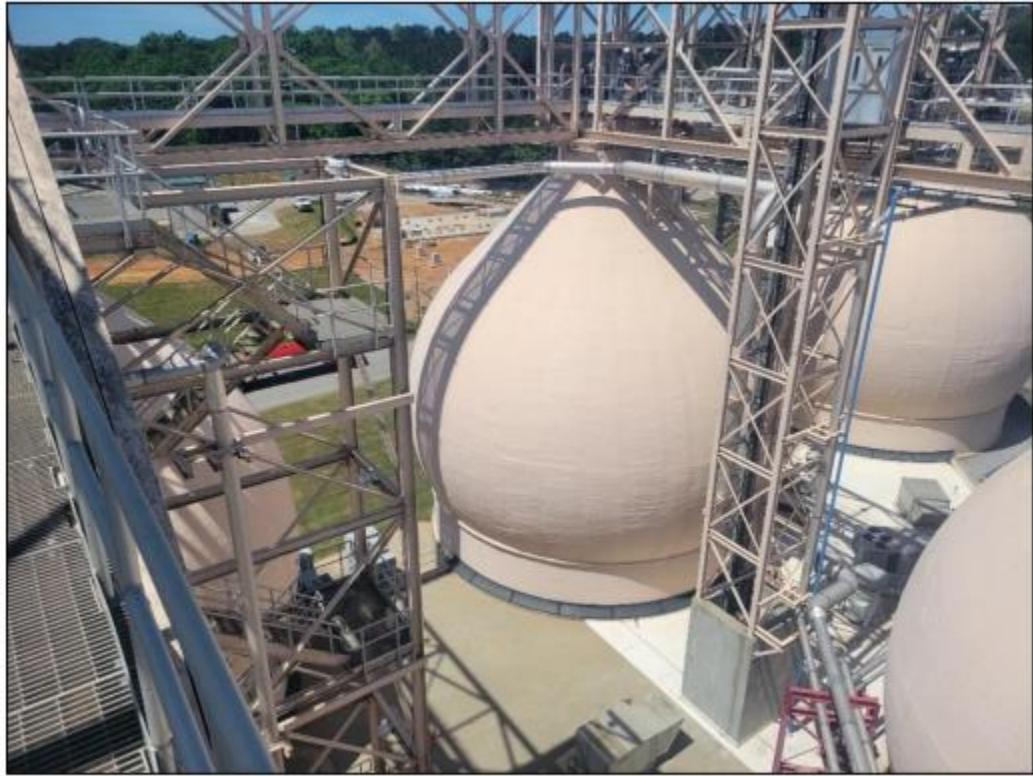
Figure 6: View of elevator tower between Digesters 4 and 5 and staircase pictured on the left.
