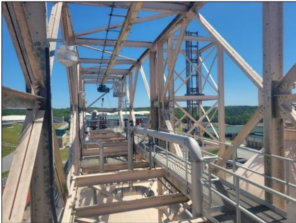
Figure 8: View of catwalk and crane rail looking towards Digester 5.
