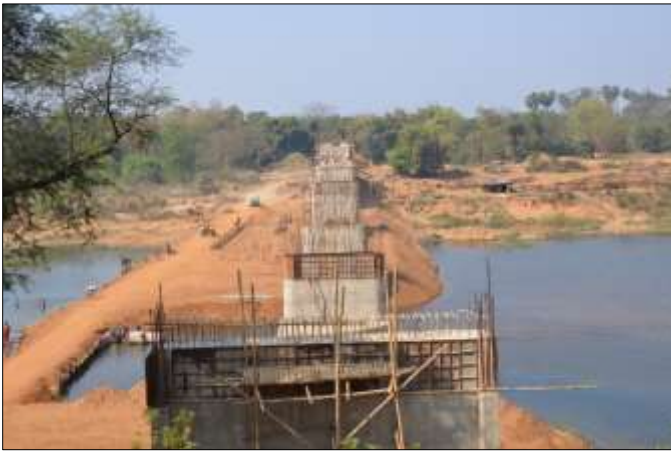
Fig. 4. Road-over-bridge construction cutting through the Budhabalanga River near Kuche (Site 4).
