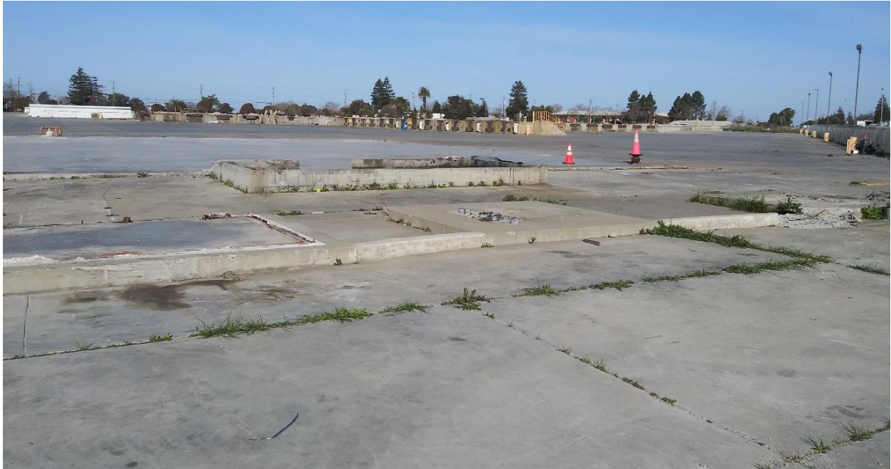
Figure 3 Concrete Surface and Building/Structure Foundations, View to the Northwest
