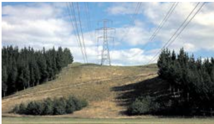
Electricity transmission lines require consideration when planting trees. These high-tension lines cross the Dolbel Estate beside Puketapu Road. Source: Kevin Thomsen
