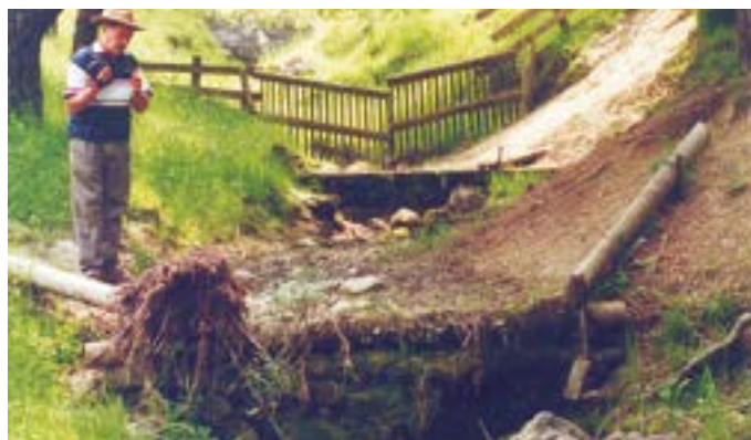
Looking underneath Pearson’s gully planting, this is what debris dam construction looks like in an eroding gully which has been backfilled with sediment. Source: unknown
