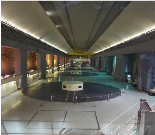
Location where the plant will be rehabilitated (REABSUL2)
