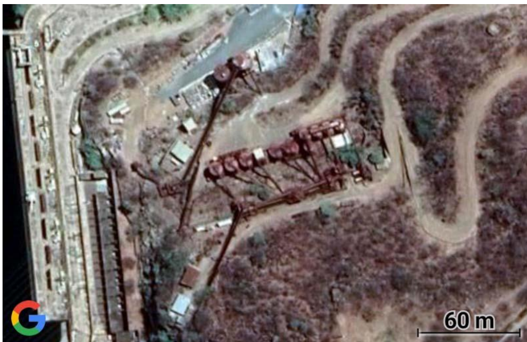
Figure 0-5 - HCB- traces of infrastructures from the time of the construction of the dam.
