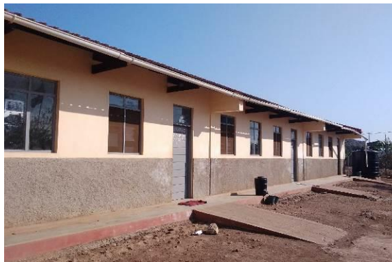
Full Primary School at Unidade Neighbourhood
