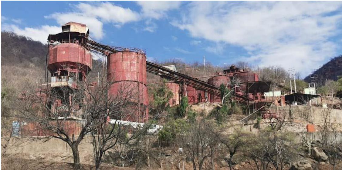
Figure 0-6 – Old concrete plant and quarry.
