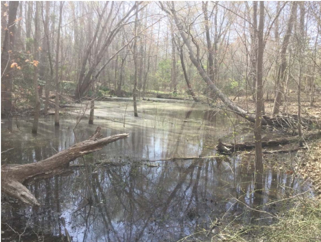
Photograph 6: View in April of VPP, a stream fed pool with a partially blocked culvert at Reynolds Drive.
