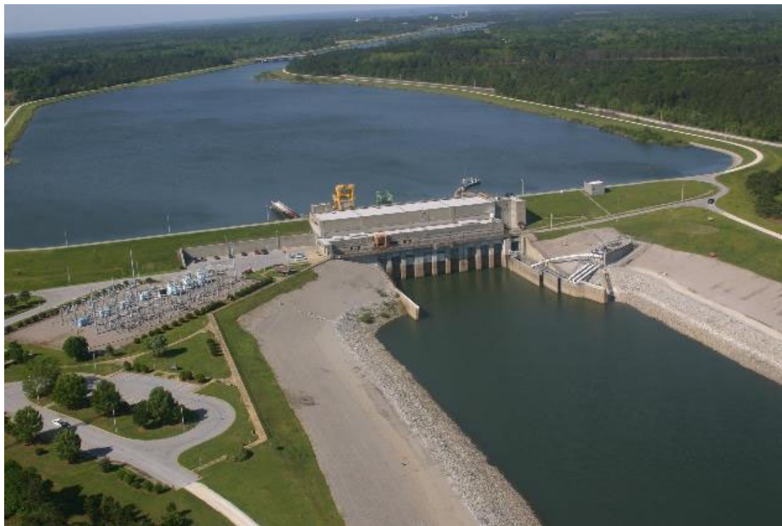
Figure 7. Cooper River Rediversion Project (USACE photo).
