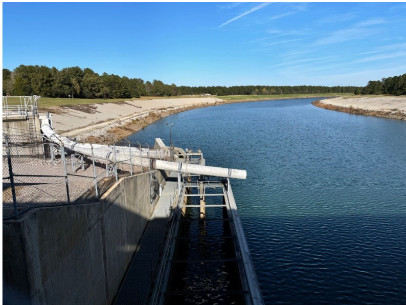
Figure 8. Fish lift at the St. Stephen Powerhouse (Lucia Wimberly, USACE, Charleston District).
