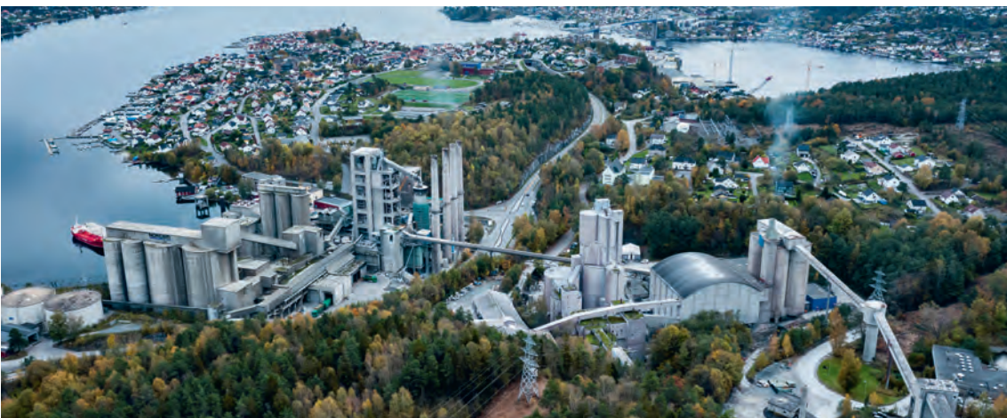
At the cement plant in Brevik, Norway, the first industrial-scale carbon capture facility is built, 2022. Photo: Dag Jenssen
