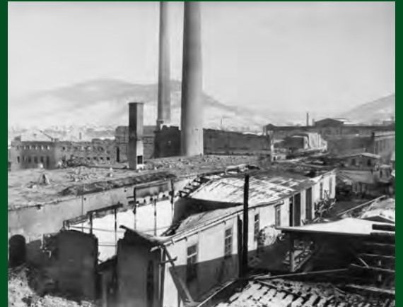
Ring kiln III in the foreground behind the shed, raw mill building on the left behind it, cement storage and shipping hall at the back on the right
