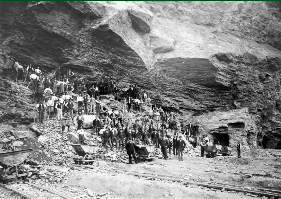
From 1879, the Rohrbach quarry on the district boundary with Leimen was operated by the company itself. The Rüdersdorf "fall operation" method was the chosen mining technique, 1895.
