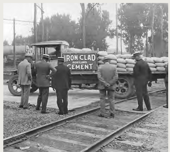
Loading test on a concrete road with a truck loaded with 6.5 tonnes of cement at Glens Falls, New York, 1929
