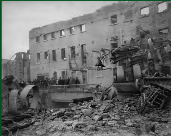
Raw mill building, in front of it a pan grinder for pre-crushing
