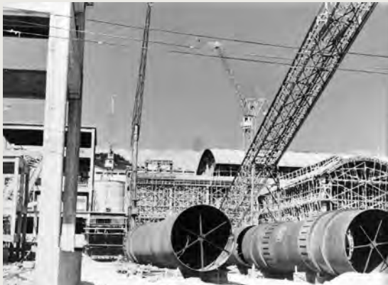
Construction of a cement plant in Monselice, 26/07/1958
