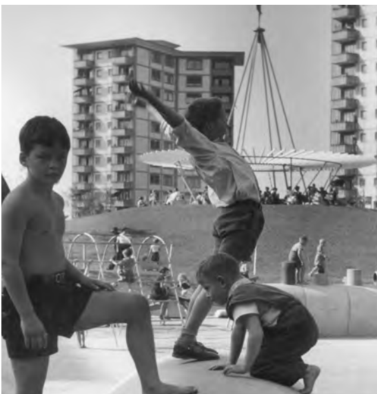
Fair-faced concrete construction with playgrounds made of concrete, circa 1965
