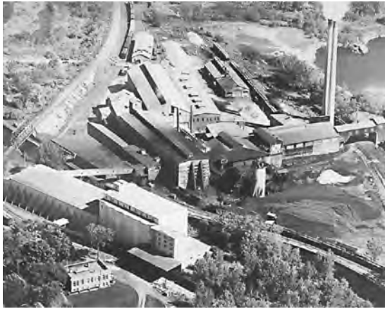
Glens Falls Portland Cement Company. The plant is now one of Heidelberg Materials' oldest still in production, circa 1967.
