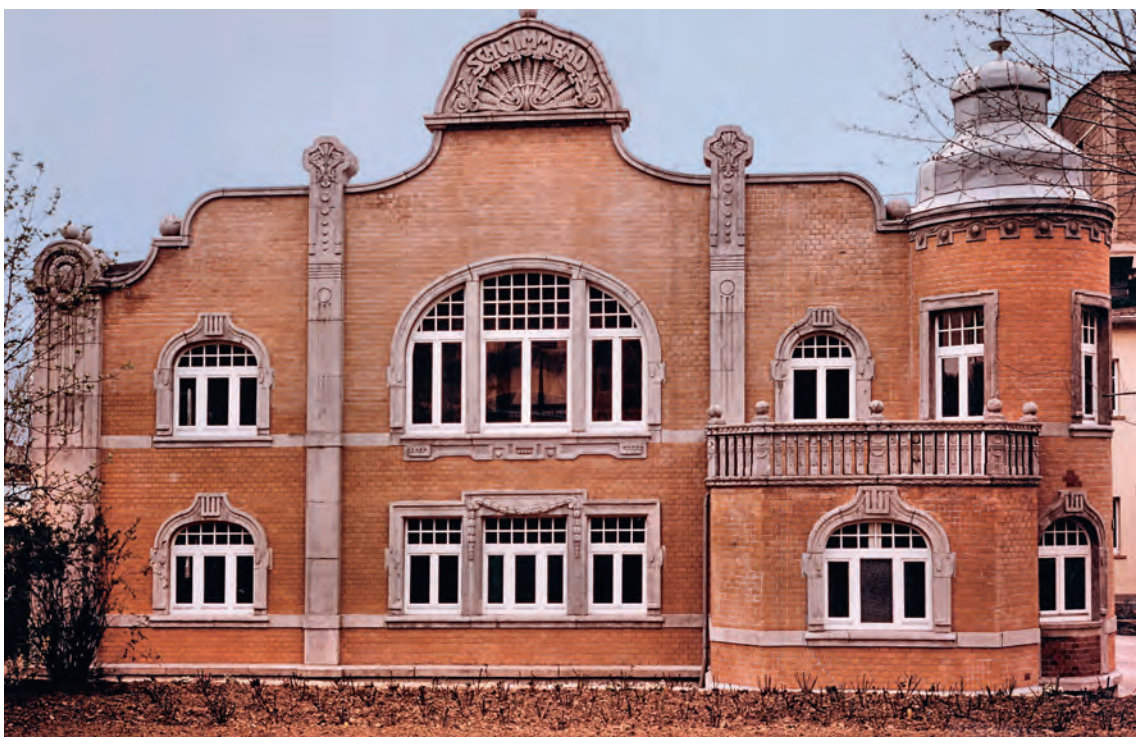
Indoor swimming pool. The 600 m 2 building is made of imitation limestone and reddish-yellow facing bricks. The pool attendant was housed in the annex with a balcony. The adjacent staircase tower led to the bath, 1983.
