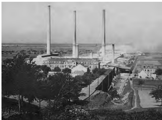
View from the east overlooking the new plant. On the left, the seventh ring kiln erected in 1898. In the foreground, the covered dumper railway flyover, 1900
