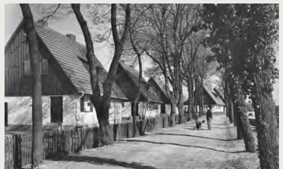
Housing development. Dr Friedrich-Kirchhoff housing estate in Weisenau, 1936
