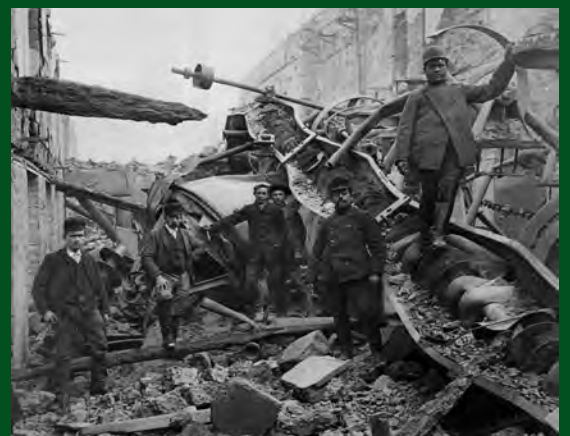
Workers in the old steam-powered cement mill
