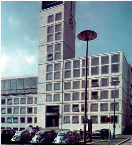
Stuttgart Town Hall designed by Hans Paul Schmohl and Paul Stohrer. Building using concrete from the Nürtingen cement plant, inaugurated on 4 May 1956
