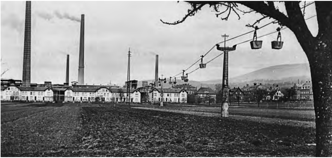
Cable car system from Leimen to Nußloch. The workers' houses at Zementwerkstraße, built in 1908, can be seen in the background, 1920.
