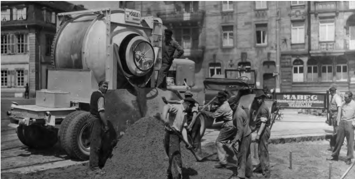
Labour service in Mannheim with one of the first Vögele ready-mix trucks in the background, circa 1935
