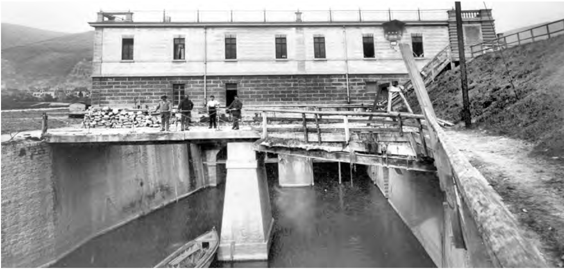
Former mill building at the Bergheim Mill. After the installation of new turbines, it had an output of 500 hp. Now the clubhouse of rowing society Rudergesellschaft Heidelberg 1898 e.V., 1900
