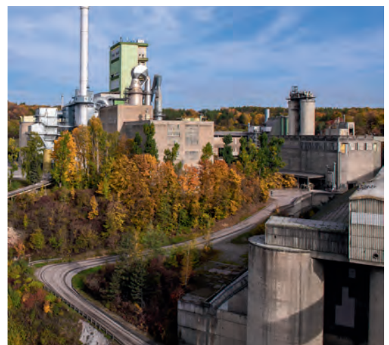
Lengfurt/Main cement plant, 22/10/2020
