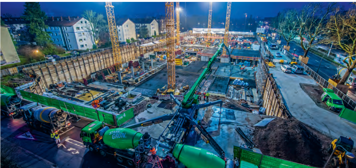
Construction work on the new headquarters, 16/12/2017. Photo: Steffen Fuchs
