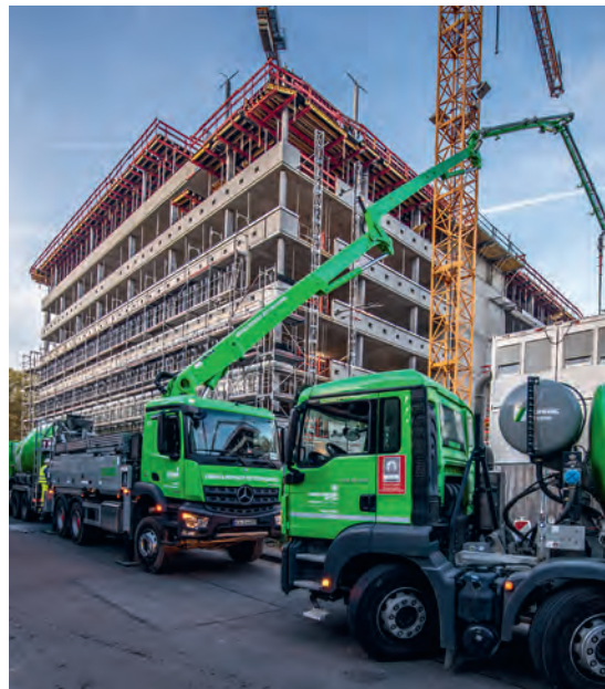
Concreting of the 5th upper floor, 18/10/2018. Photo: Steffen Fuchs
