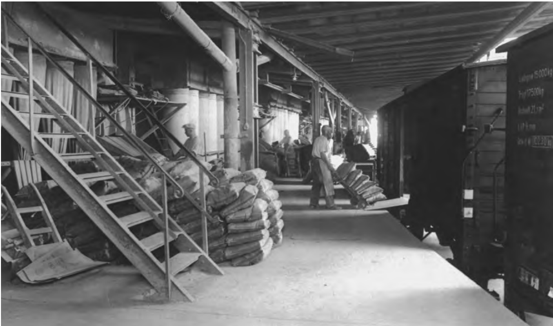
Loading sacks into railway wagons in Leimen, 1935
