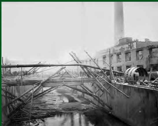
Mill race with the cement mill building on the right
