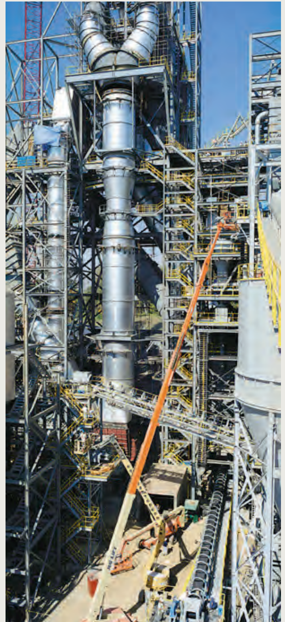
Preheater kiln under construction at the Union Bridge plant, 2002
