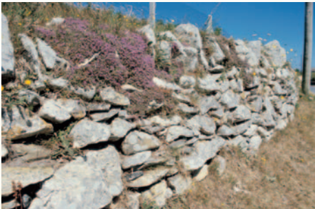
Retaining wall ( L.Lysaght )
