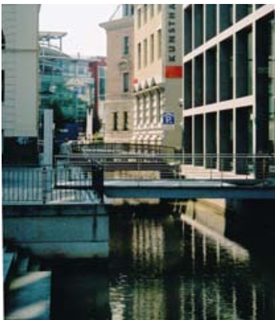
New footbridges link waterside walkways with new or redeveloped property. © Roger Butler
