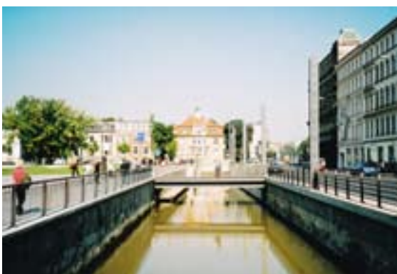
Newly rebuilt navigation close to some of Leipzig's historic landmarks. Works include access to pontoons, footbridges, artwork, lighting and improved civic spaces linking to the main canalside routes. © Roger Butler
