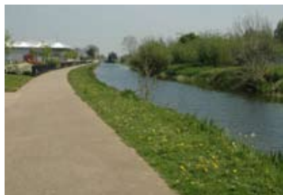
New spray and chip towpath on the Royal Canal at Ashtown, with substantial soft edge. © Roger Butler
