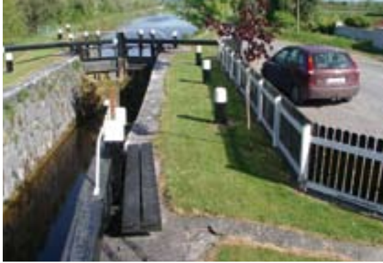
Grass surfacing at lockside incorporating mooring bollards. © (Colin Becker)
