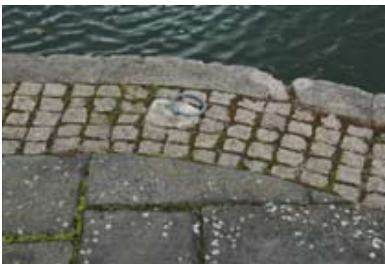
Towpath treatments at the restored Market Harborough Basin, with granite setts providing a trim to the water's edge and stone flagstones marking the main pedestrian walkway around this part of the basin © Roger Butler
