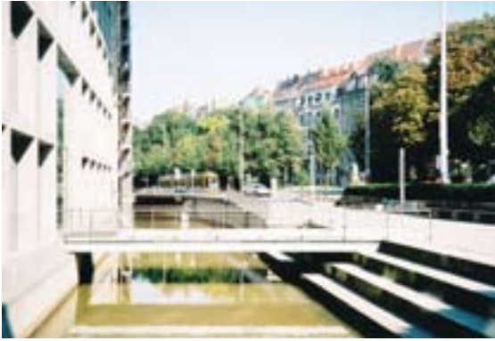
Formerly culverted waterway opened up for public use. New footpaths and pedestrian bridges link offices, apartments and open spaces © Roger Butler
