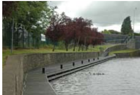
Timber pontoon and access ramps for water polo and canoe launching, © Roger Butler
