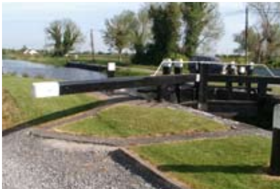
Hard surfacing for heel grips in arc of balance beam. © (Colin Becker)
