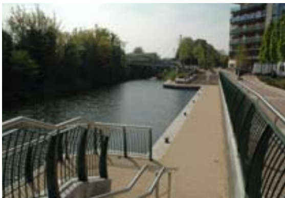
A new mooring lay-by with public access from the towpath has been created as part of the Ashtown development at Lock 10 on the Royal Canal. © Roger Butler
