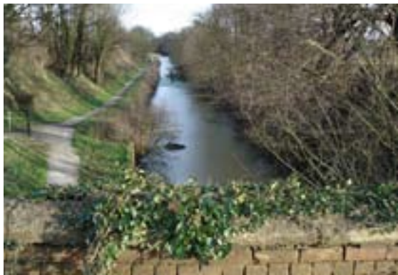
Rural towpath on the Grantham Canal, improved with limestone surfacing to provide access along a popular length of the waterway © (Roger Butler)
