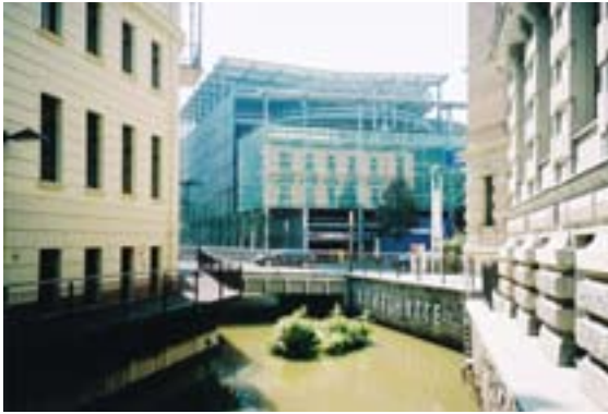
Cantilevered walkways installed to enable continuous public access in confined areas. Ecological works encourage aquatic planting and artistic work in the form of wording which reflects in the water. © Roger Butler
