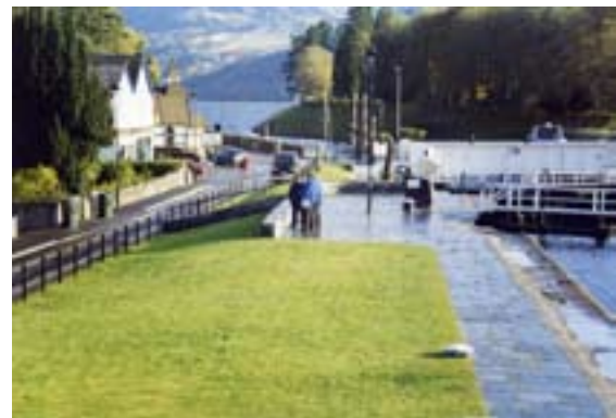
Fort Augustus lock flight after major landscape improvements, including new Caithness flagstone paving, new access points, seating and lighting. © Roger Butler
