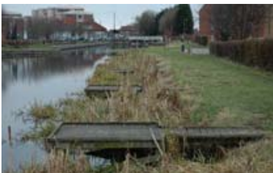
An offside path enabled easily accessible fishing platforms to be installed on the opposite side to the towpath, helping to prevent conflict between different towpath users. © (Roger Butler)
