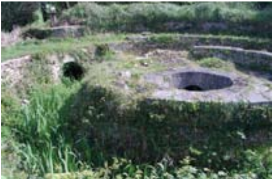
The Four Pots. A disused overflow system, near Digby Bridge, Grand Canal, Co. Kildare. © (Colin Becker)
