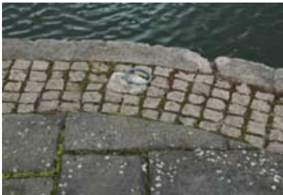
Towpath detail at Market Harborough Basin, with waterway copings, granite setts and stone flagstones © Roger Butler
