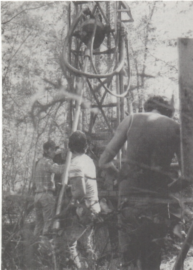
Drilling of shot hole.
