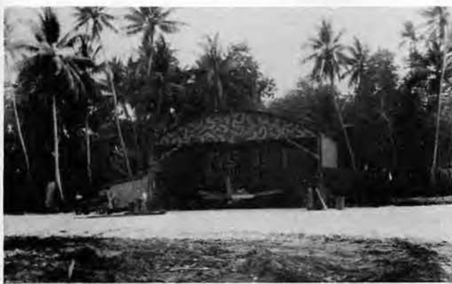
ONE OF THE AIRCRAFT repair hangars constructed by 16th Seabees for Marine and Army fliers at Island "X" is shown in above photo. Seabees machinists often assisted air corpsmen install new motors in heavy Liberator bombers.
