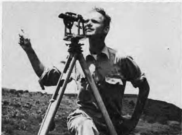
THE LARGEST SINGLE, major construction job assigned the Sixteenth Battalion in Hawaii was the erection of a Naval Supply storage area. This task was undertaken in Feb. 1943. Surveyor Durlinger is shown above "shooting angles" for the roadway.
