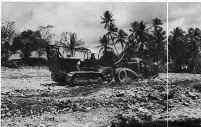
TRACTOR AND CARRYALL shown in foreground are grading foundation for bomber strip. Equipment of this type roared continually day and night to complete the vital air strip in record time.
