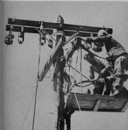
LINEMEN AT WORK
