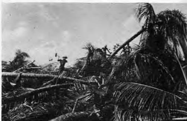
WHEN THE TOWERING palms were uprooted and felled to the ground, Seabees moved in with axes. Men assigned this job had to work fast for bulldozers, carryalls and cranes were standing by to clear the debris for the proposed bomber strip.
