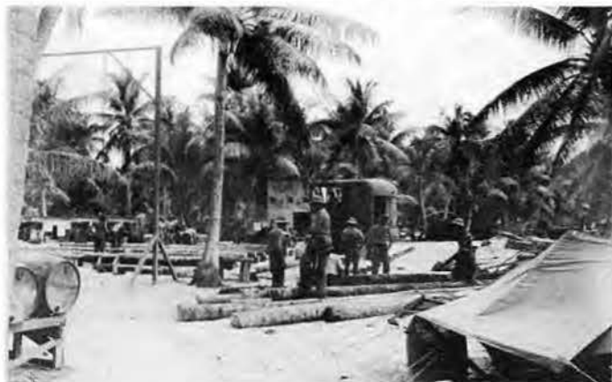
NEXT TO A HUGE mail delivery with plenty of letters from home—movies—good bad or indifferent ranked No. 1 as a morale builder on Island "X." 16th Seabees are shown above constructing open air theater on Nanumea.
