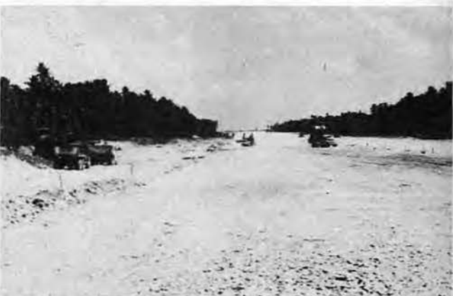
IN THE FOREGROUND, picture shows clearly the large rock used as foundation for bomber strip. Over this was rolled layer upon layer of glaring, snow-white coral. Ten-ton rollers packed the coral as hard as concrete highway.
