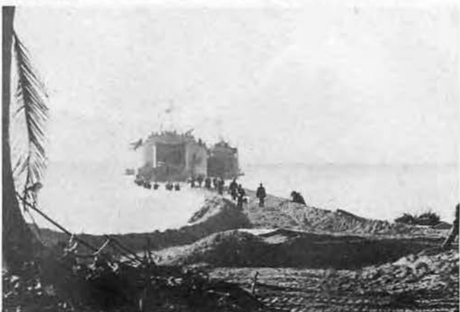
COCONUT LOGS were used for "cribbing" and foundation for the road. Crews assigned to this detail often worked during high tides.
