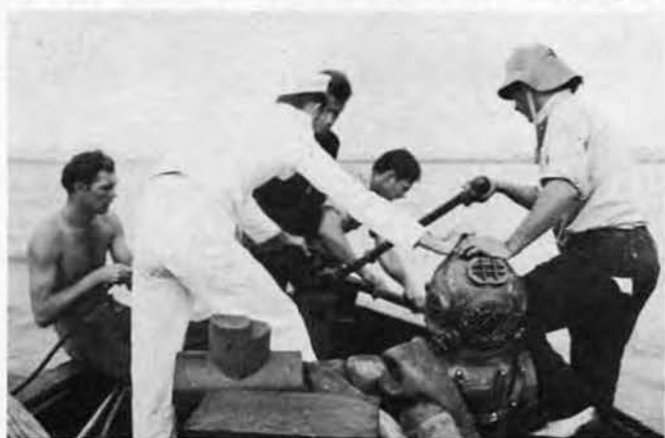
ARRIVING AT THE PROPER depth required for the final rigid examination, 16th Battalion divers lower heavy anchor. The same men pictured here later helped raise the USS Oklahoma.
