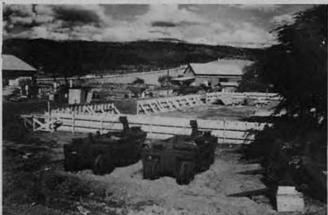
IN CENTER of picture beyond carryalls in foreground can be seen the foundation for the second large warehouse.
