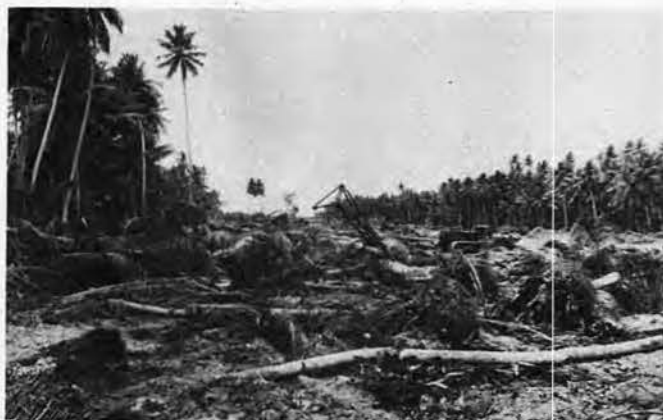
NEARLY 50,000 TREES were knocked down when this picture was made. Rig in the foreground was used to load roots on trucks. The island was so small, much of this debris had to be thrown into the ocean to conserve space.
