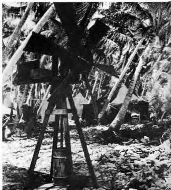
INGENIOUS SEABEES constructed various novel washing machines from spare parts and scrap lumber at Island "X." The one shown above worked efficiently—when there was a strong breeze.
