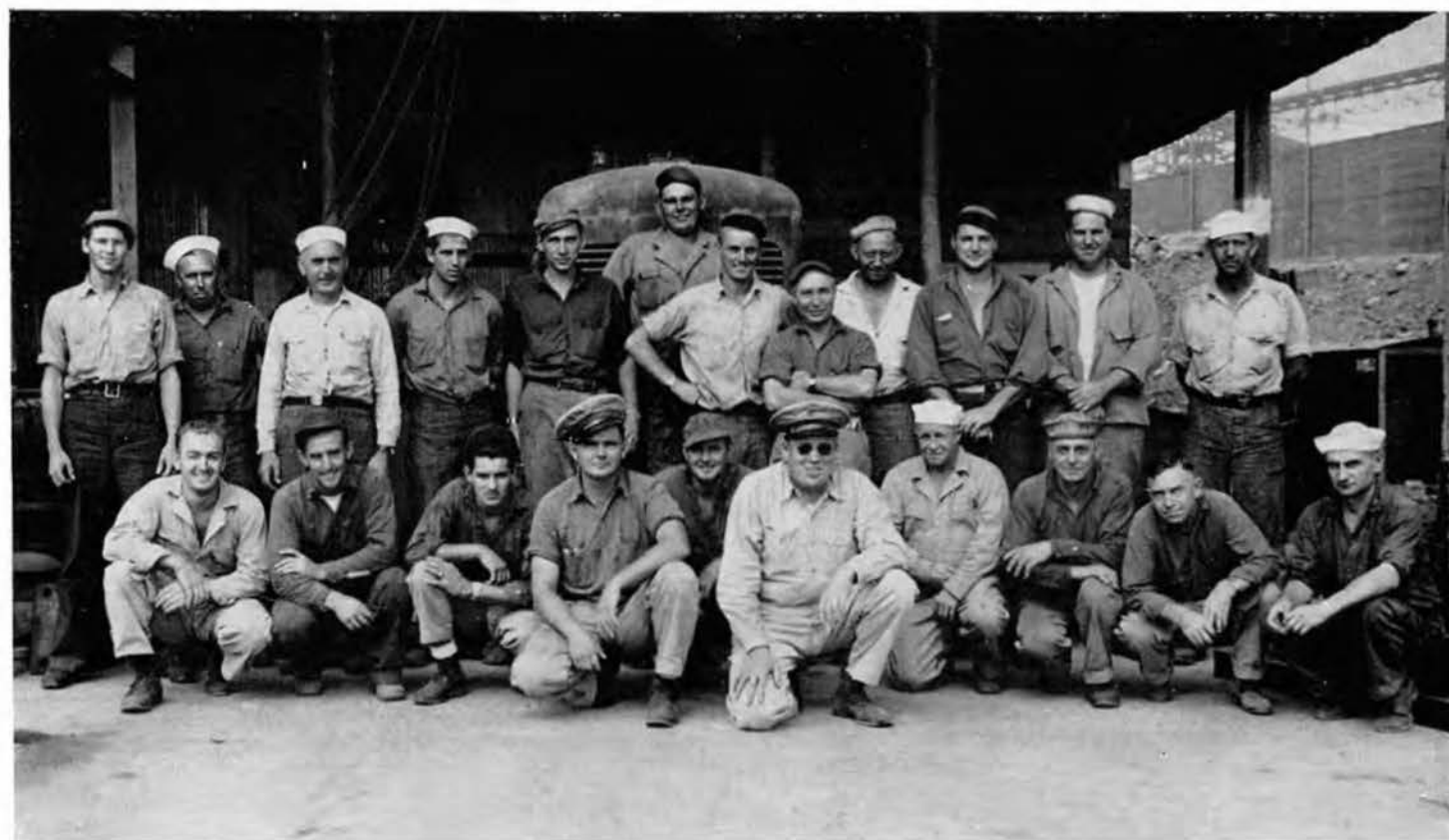
HEAVY EQUIPMENT REPAIR
