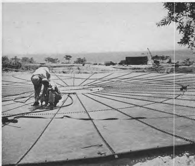
Seabees prepare foundation for fuel tank — one already completed is shown at right.
