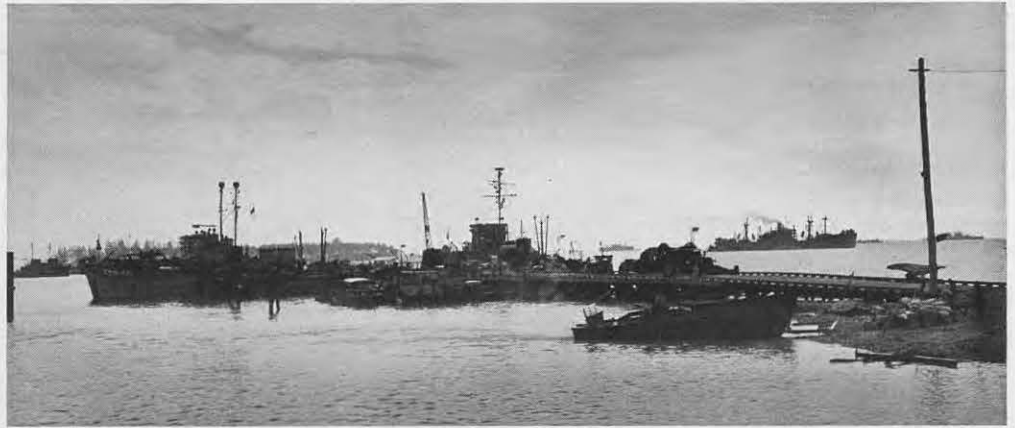
Completed timber pier replaces pontoon dock destroyed by storm.
