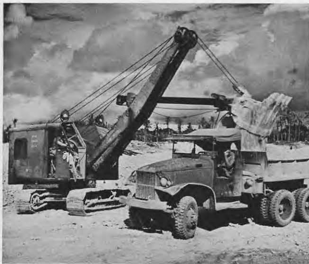
Loading coral for surfacing hardstand (see right).
