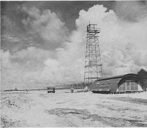
Finishing work on control tower structure.
