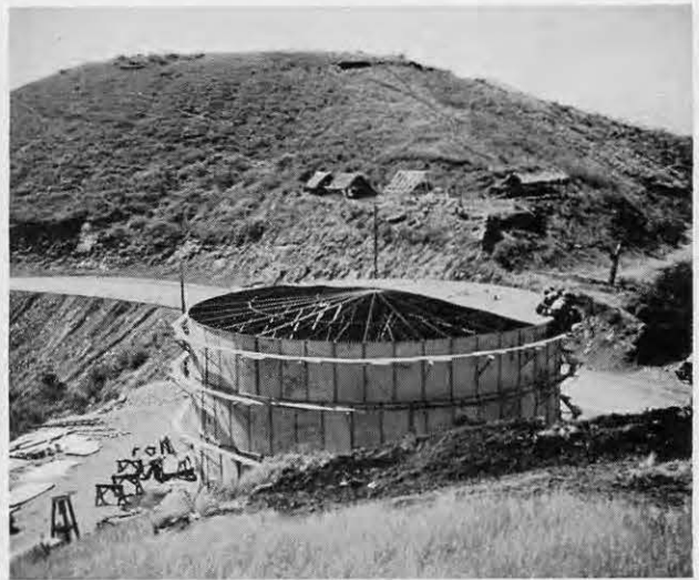
Near completion of water storage tank.
