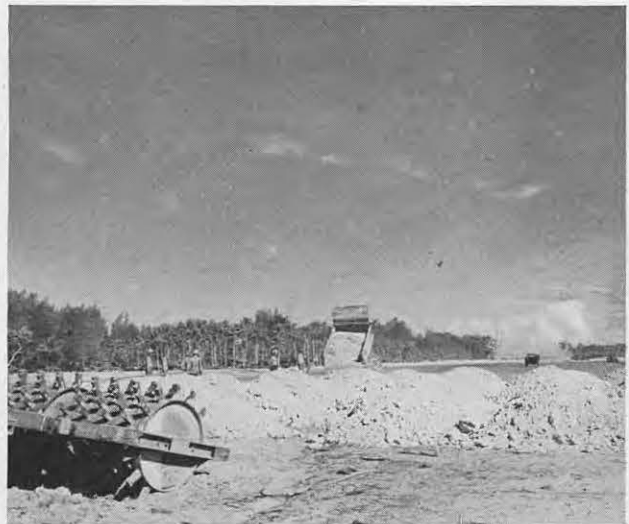
Dynamite loosed coral rock loaded on truck for delivery to fast-taking-shape airstrip.
