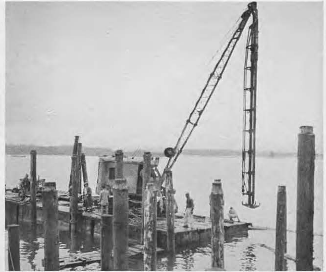
Timber pier under construction.
