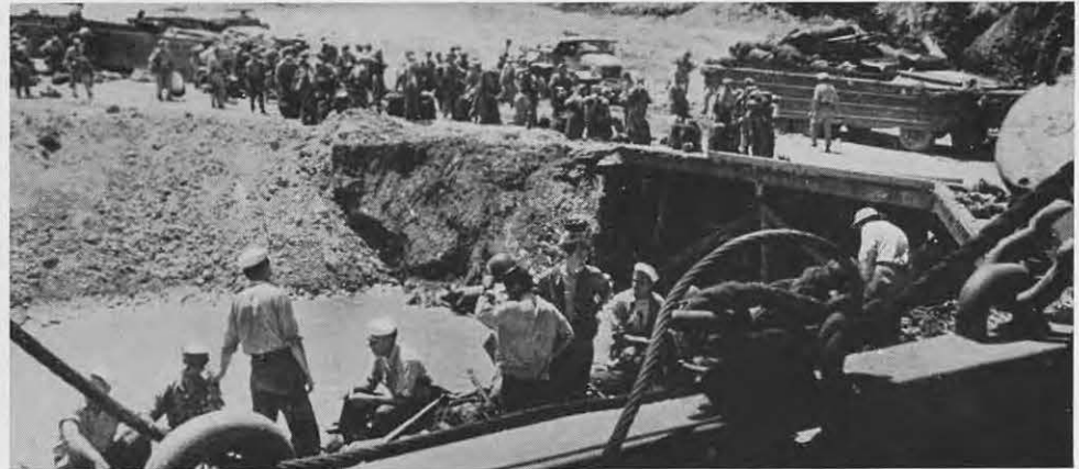
Seabees have pier completed for arrival of echelon.
