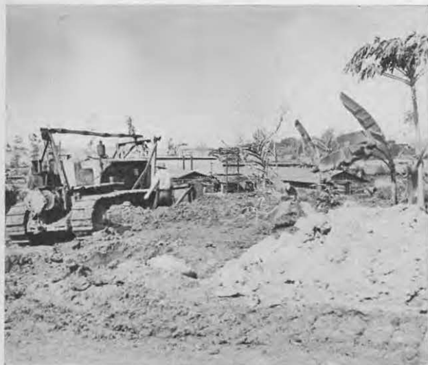
Leveling ground for construction work.
