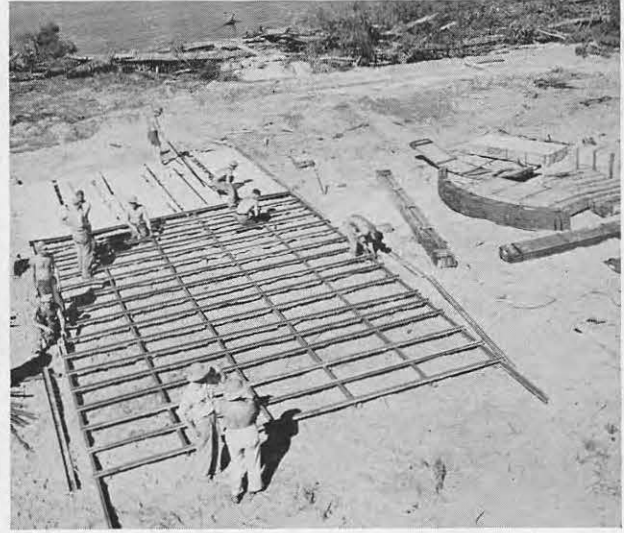
Preparing deck for parking area workshop.
