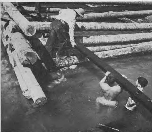
Coconut cribbing for floating dock approach.
