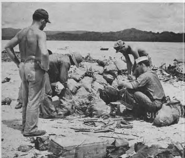
Scores of dynamite laden burlap bags prepared for coral blast — depicted so picturesquely at right.
