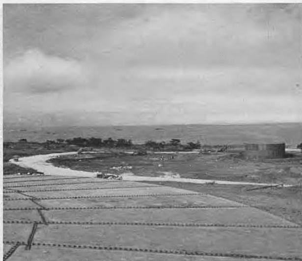
Seabees prepare foundation for fuel tank — one already completed is shown at right.
