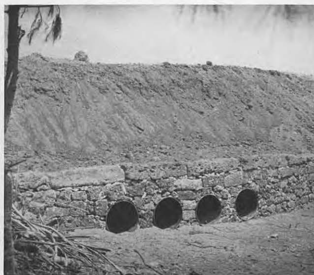
American pipe and native stone combined in making a durable drainage culvert.
