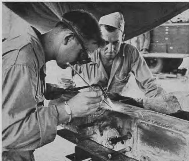
Welding 'dozer water jacket hit by land mine.
