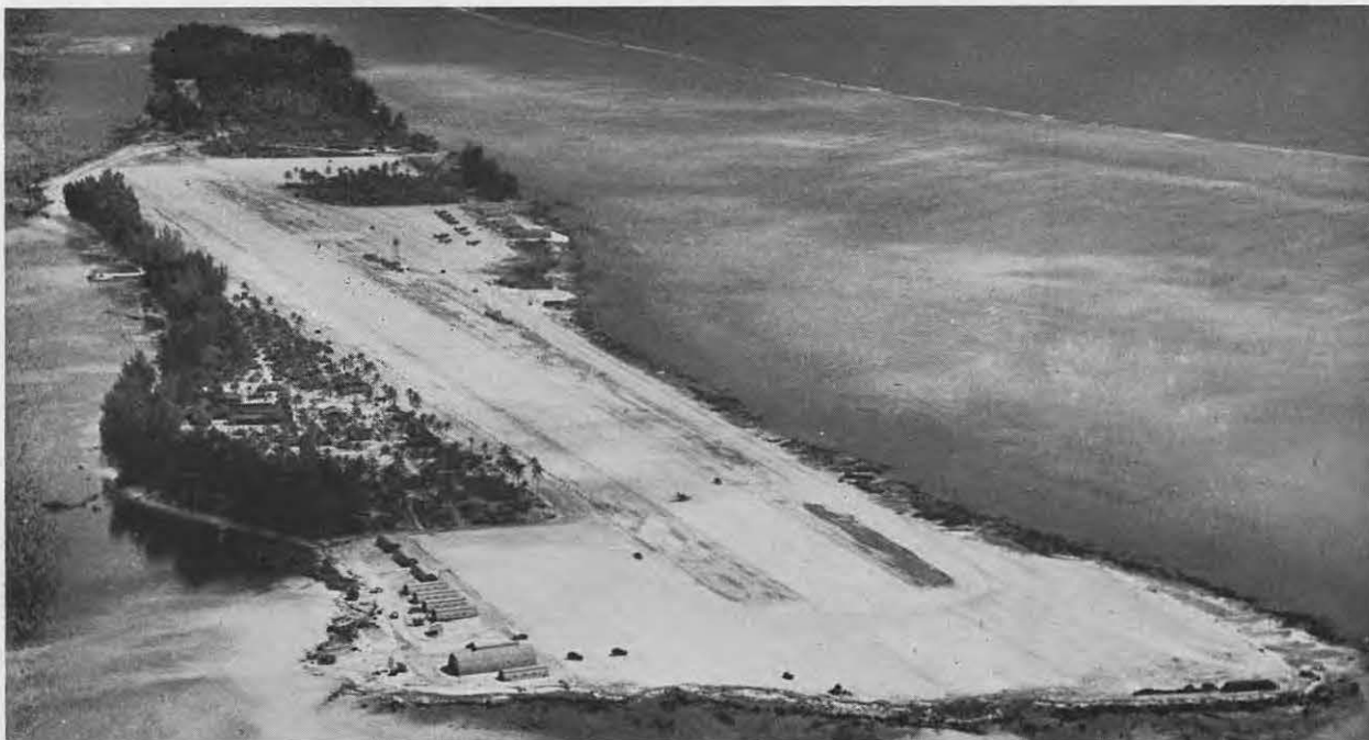
Aerial view of finished product, — note glistening coral surface, remnant of coconut plantation.
