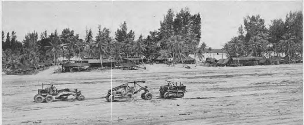
Grader rolls behind earth-mover — observe movie screen right center.
