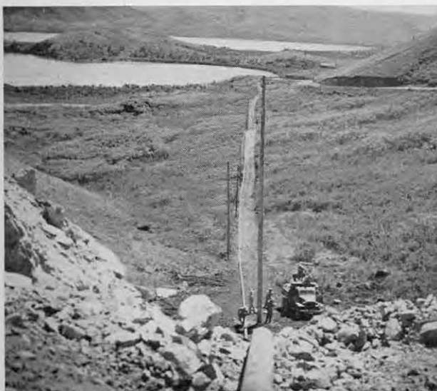
Construction of pipeline nears end.
