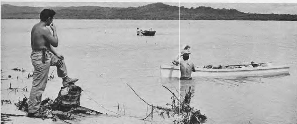
Dynamite conveyed by dory for blasting solid coral rock.
