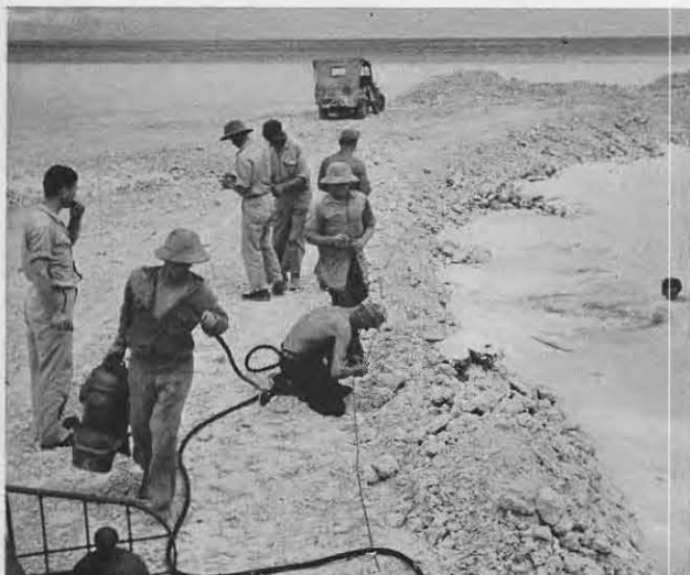
Preparing wiring for dynamite blast.
