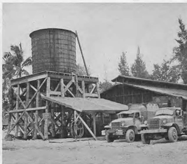
Water storage and chlorination unit.
