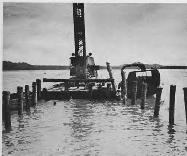
Driving piles for small craft dock.
