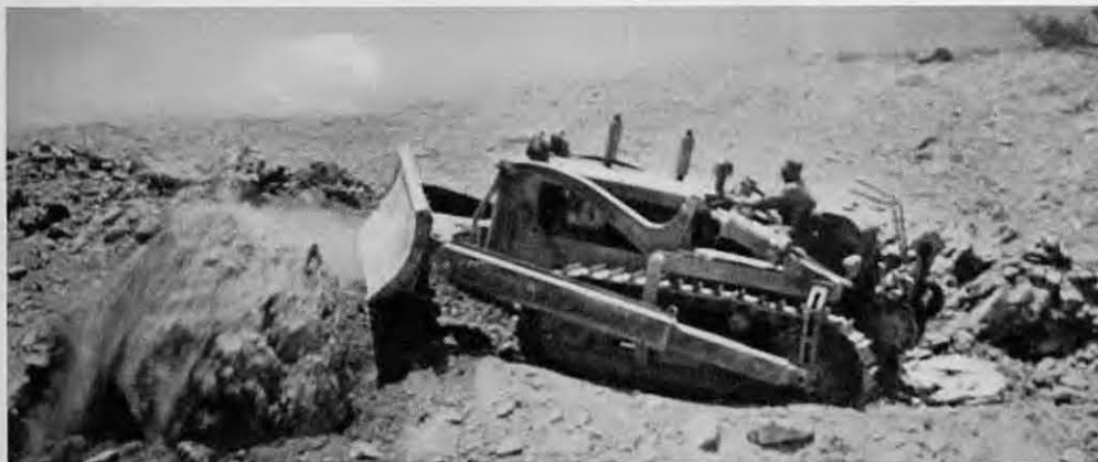
Angle dozer — bulldozing sidesaddle to clear surface for waterline.
