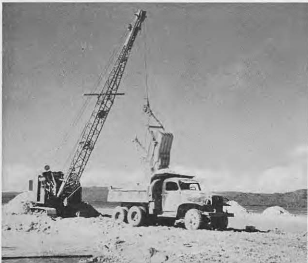
Dynamite loosed coral rock loaded on truck for delivery to fast-taking-shape airstrip.
