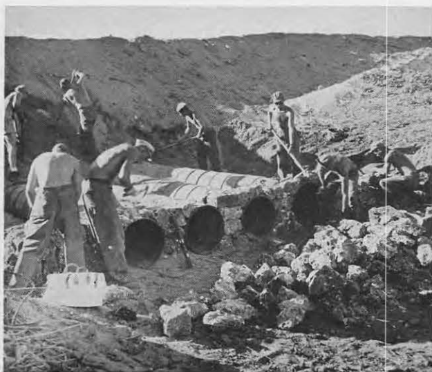
American pipe and native stone combined in making a durable drainage culvert.
