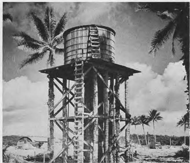
Water tower with cocoanut tree trimmings—Butjo-Lang.
