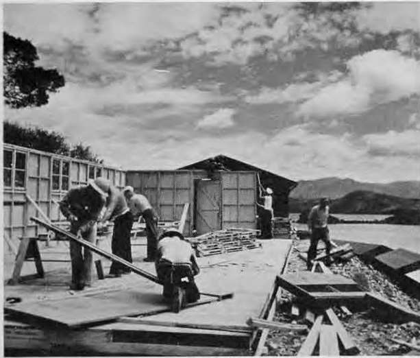
New Zealand prefabricated warehouse at Ducos.
