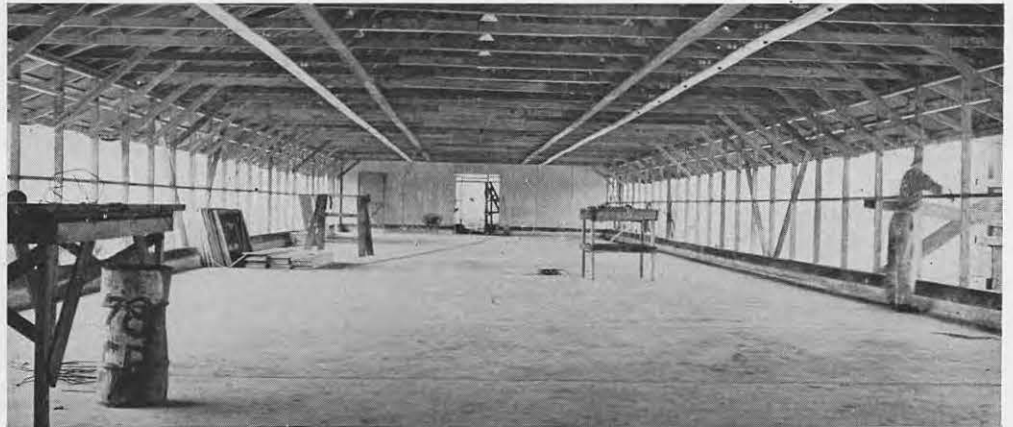
Bulkhead structure completed for screening in of Hospital Mess Hall.
