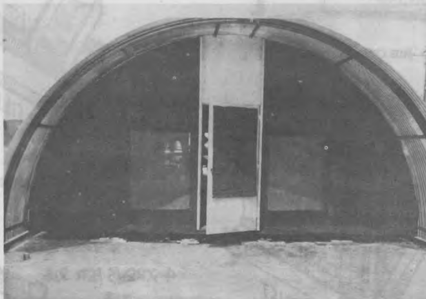
VIEW OF TROPICAL EXTENSION AND BULKHEAD
