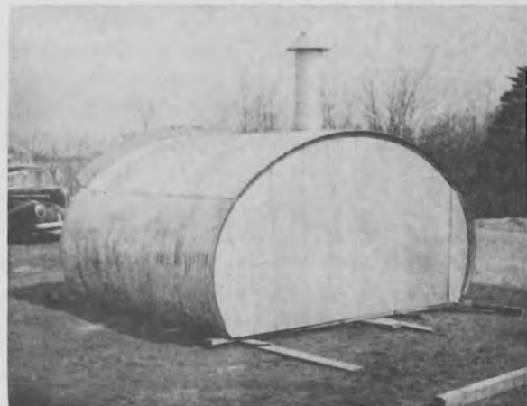
EXTERIOR REAR VIEW
