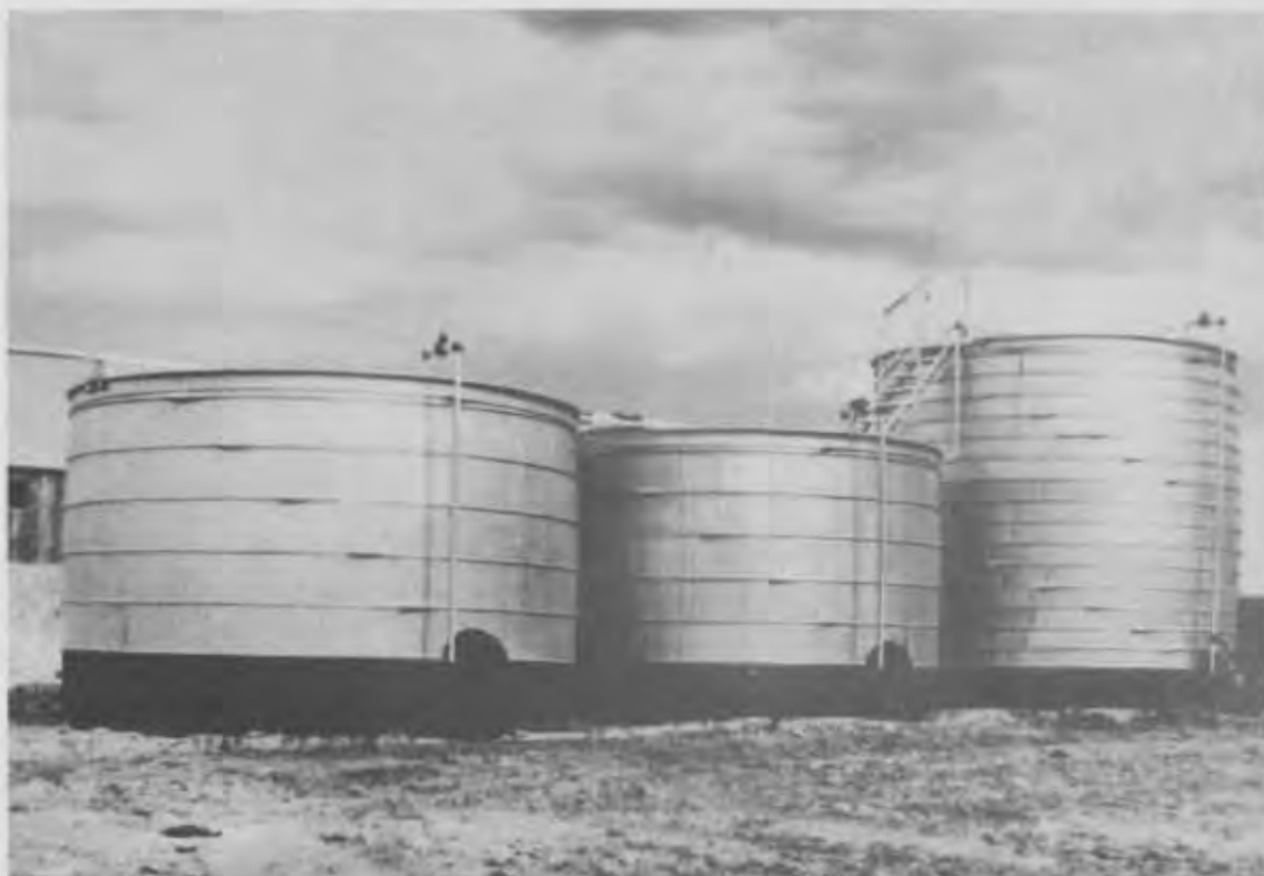
WOOD WATER TANKS (2H71)
