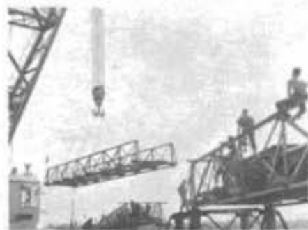
MCB-FIVE Charlie Company pendant flies from new bridge section being installed on Tourane (Da Nang) River bridge by a floating crane.
