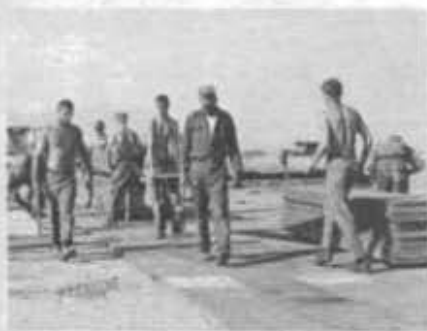
Seabees of MCB4 rehabilitate "the Chu Lai Funway"
