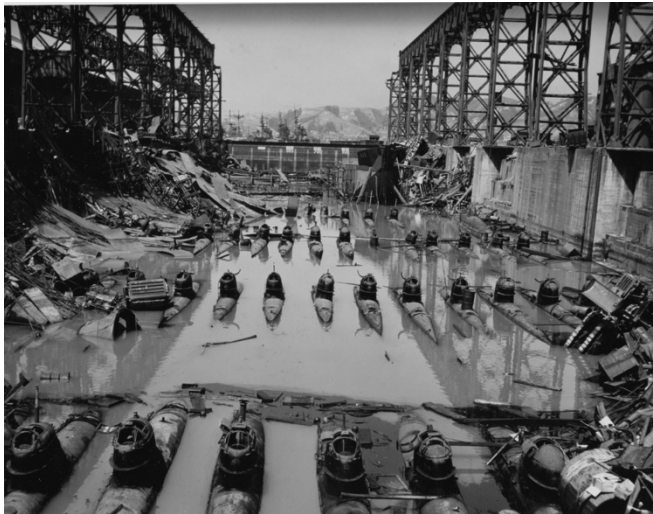
Japanese Type D (Koryu) midget submarines in a partially flooded dry dock at Kure Naval Base, Japan, February 1946. The larger vessel in the drydock, right background, appears to be a barge. Flooding, deposit of debris (including a bulldozer) and other damage was done after mid-October 1945. Official U.S. Air Force photograph. (USAF K-6023)
