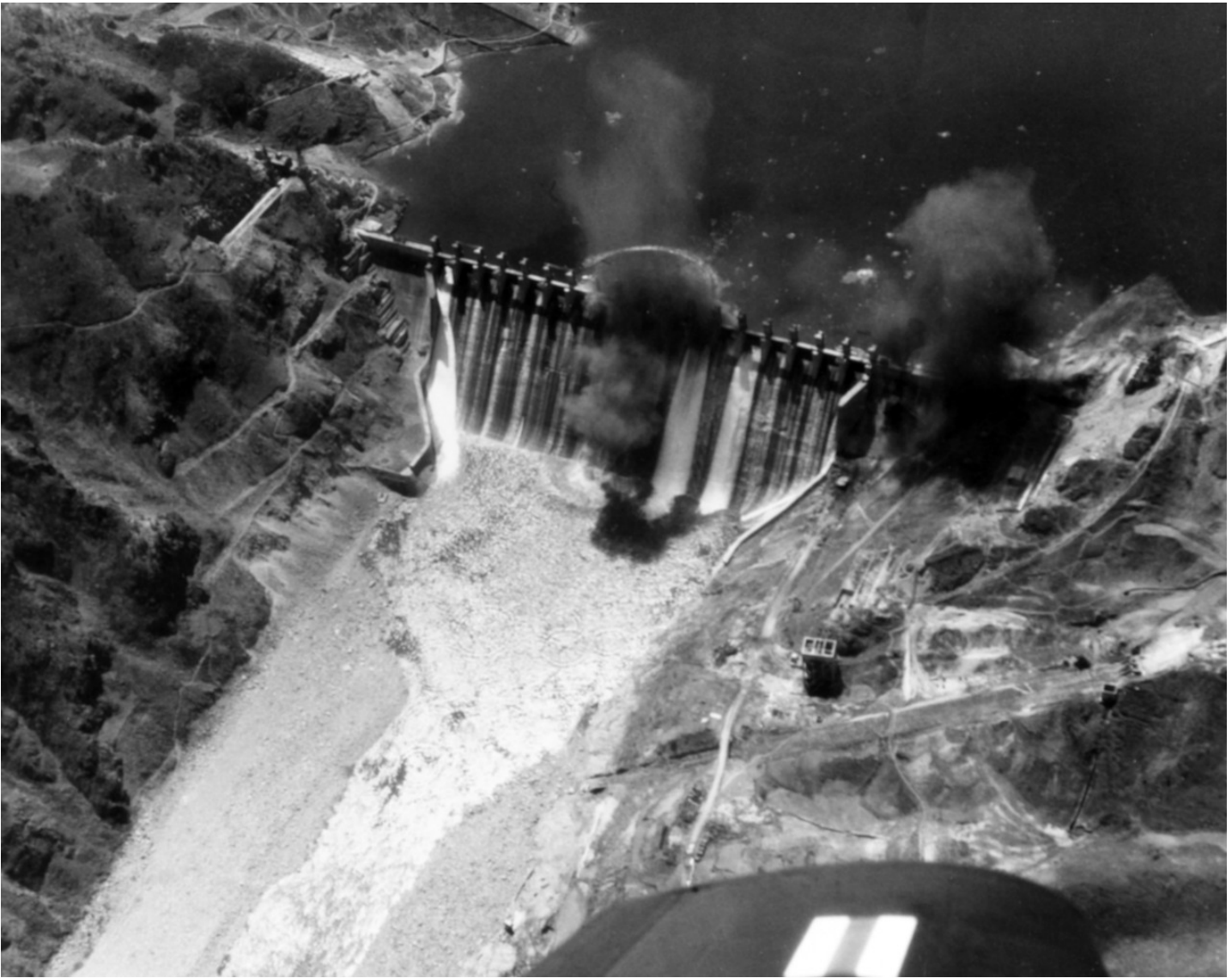
Torpedo attack on the Hwachon Reservoir dam by AD Skyraiders of Attack Squadron 195 (VA-195) from USS Princeton (CV-37), 1 May 1951. This successful strike, and earlier bomb attacks by Navy and U.S. Air Force planes, were made to deny the enemy the tactical use of controlled flooding on the Pukhan and Han rivers. Torpedoes were used after bombs failed to achieve the desired results. They destroyed one flood gate and partially destroyed another. This was the only Korean War use of aerial torpedoes. The Hwachon Reservoir was later recaptured by UN forces (80-G-428678).
