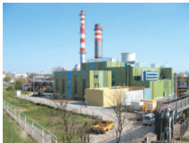
Fig. 9—NYKCE Project of E.ON Hungária in Hungary. This power plant was constructed to supply power to nearby factories through a grid interconnection while also supplying heat for space heating.
