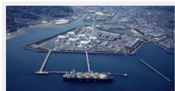
ACC: advanced combined cycle power plant (a combined cycle power plant incorporating a high-performance gas turbine with a combustion temperature of 1,300°C)
