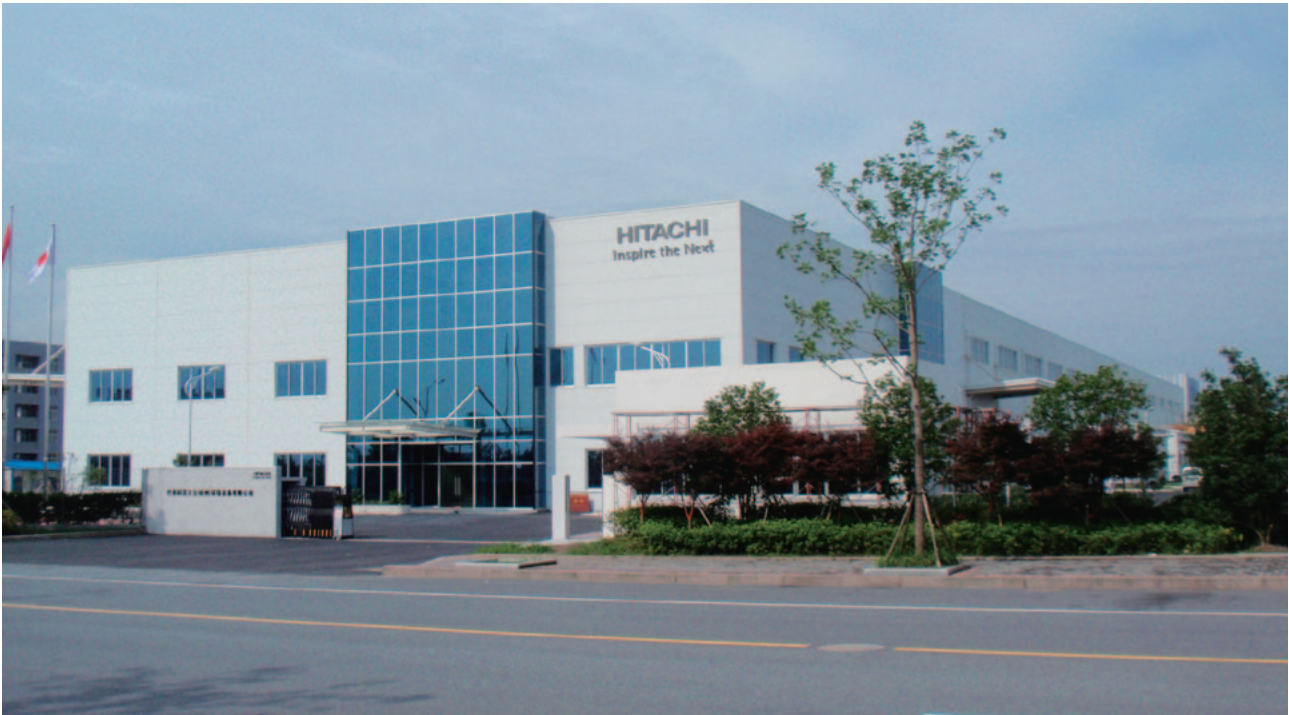
Fig. 3—Denitrification Catalyst Factory in Hangzhou, China.
