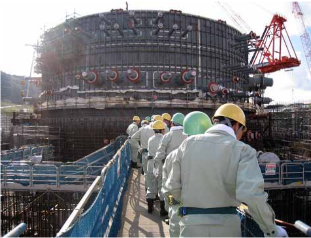
Fig. 5—Construction Site Visit.
