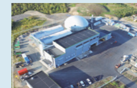
Methane fermentation facility (Biogas plants)
