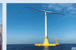
Wind power generation (NEDO Technology demonstration experiment of a next-generation floating offshore wind turbine system [barge type])
