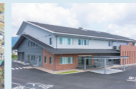
Sludge recycling center
