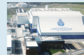
Waste to Energy plant
