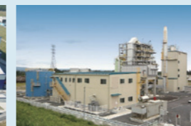
Biomass power plant
