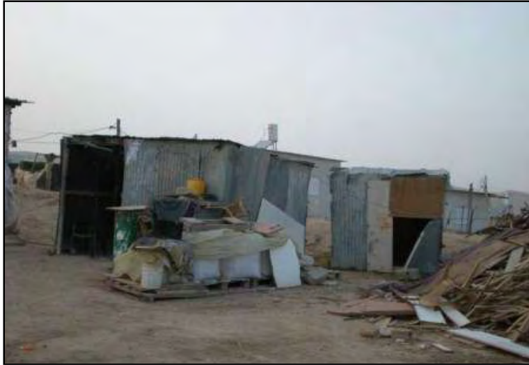
Bedouin home, al-Sirra village. All the homes in this unrecognized village are under a village-wide demolition order.
