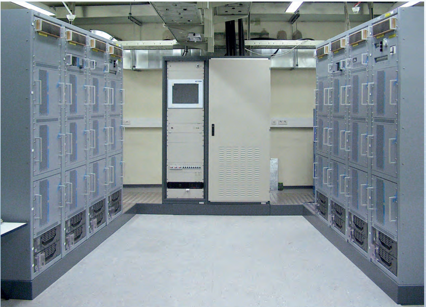
German shore station with two 10 kW HF transmitters
