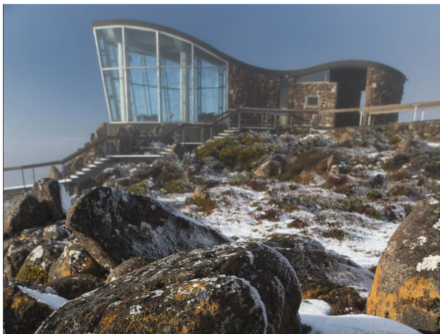
Plate 1: Existing lookout shelter, northern elevation 2
