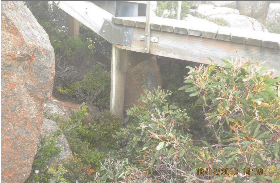
Plate 17: Vegetation growing under existing raised boardwalk
