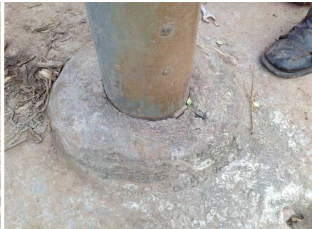
Fig. 10: Cracks at the base of a shallow well in Kalangaalo Kyamagamule
