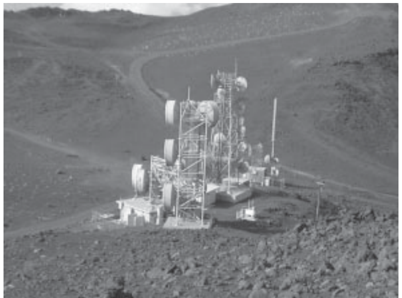
Transmitter facilities in the saddle area (Photo: Michael Maberry)
