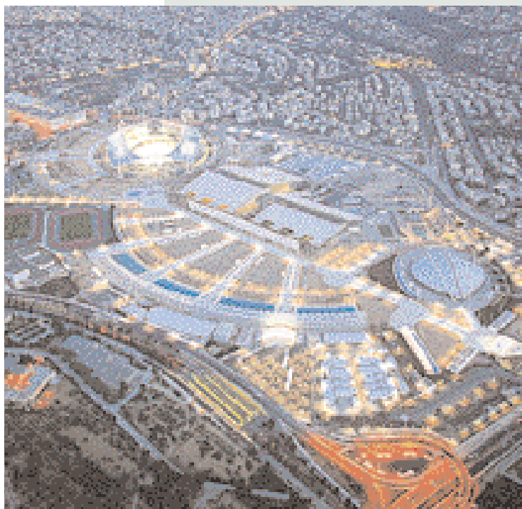
GREECE | Cement | Olympic Center (O.A.K.A.) general view for the 2004 Summer Olympics in Athens | Heracles supplied 1.4 million tonnes of cement over five years for the construction of Olympic-related infrastructure
