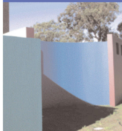
AUSTRALIA | Gypsum | Sutherland Hospital
