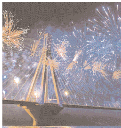
GREECE | Aggregates & Concrete | Rion-Antirion bridge, linking Peloponesos with mainland Greece | Lafarge supplied all the aggregates for its construction
