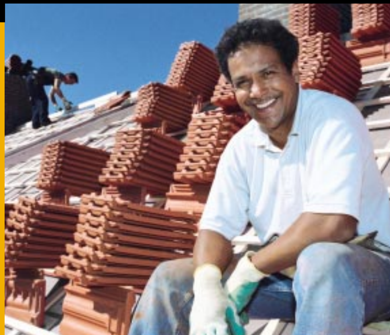
The Netherlands | Roofing | Renovation project with clay roof tiles in Oisterwijk
