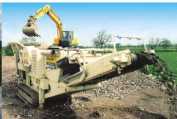
▲ United Kingdom | Crushing construction waste to preserve natural resources
