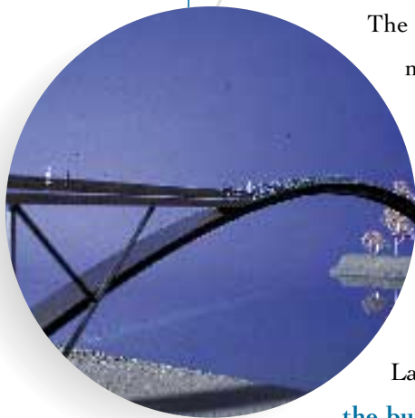
The Peace Bridge project in Seoul (South Korea): the use of Ductal® means that the deck of this future footbridge will be only 3 cm thick for a span of 120 metres
