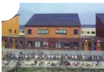
Netherlands – Solar energy panels are incorporated into the roofing of 40 houses in Amersfoort
