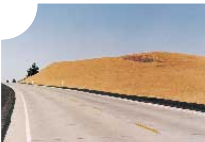
United States – Concrete road surfacing reduces fuel consumption and therefore lessens exhaust gas emissions. Pictured: Route 195
