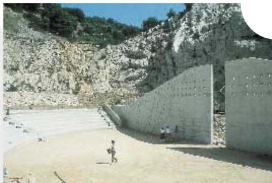
France – Concrete – The back wall of the Allauch open-air theatre, built on the site of a former quarry, was constructed with Agilia®
