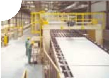
Italy – The Corfinio plasterboard plant
