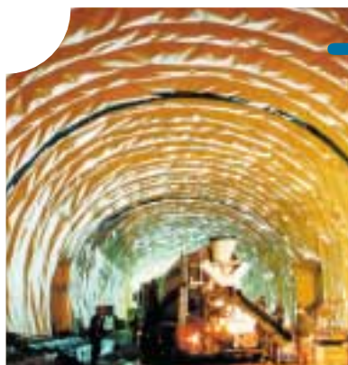
Germany – Concrete – Development of an ultra fast-setting shotcrete
