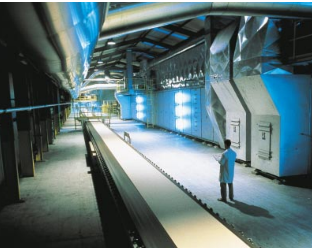
United Kingdom / The Bristol plasterboard plant.
