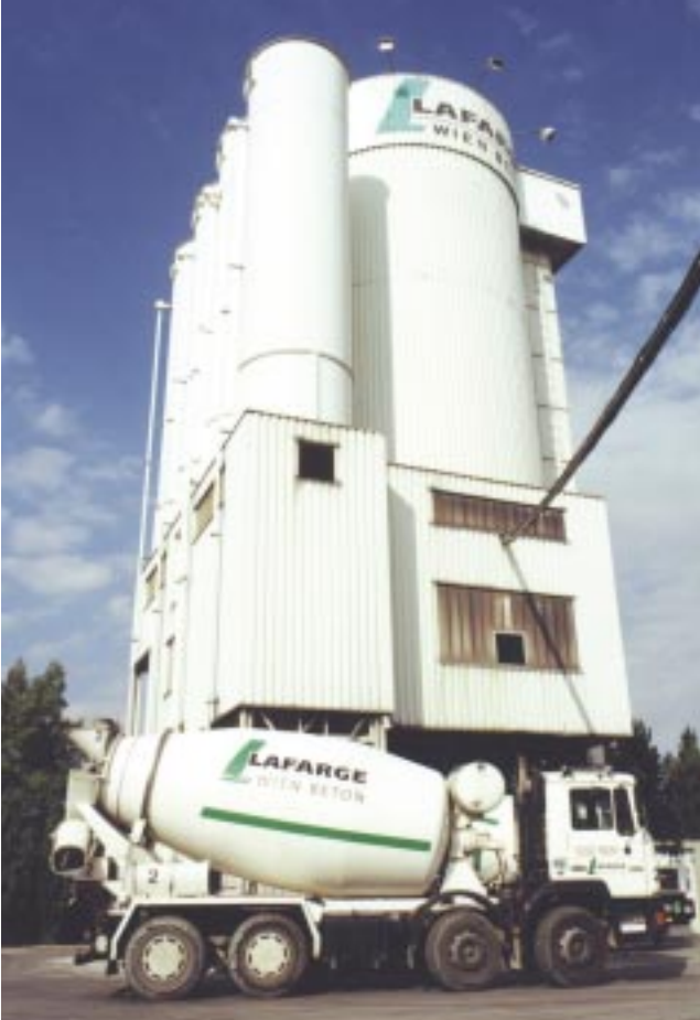
Austria / Concrete plant in Vienna.
