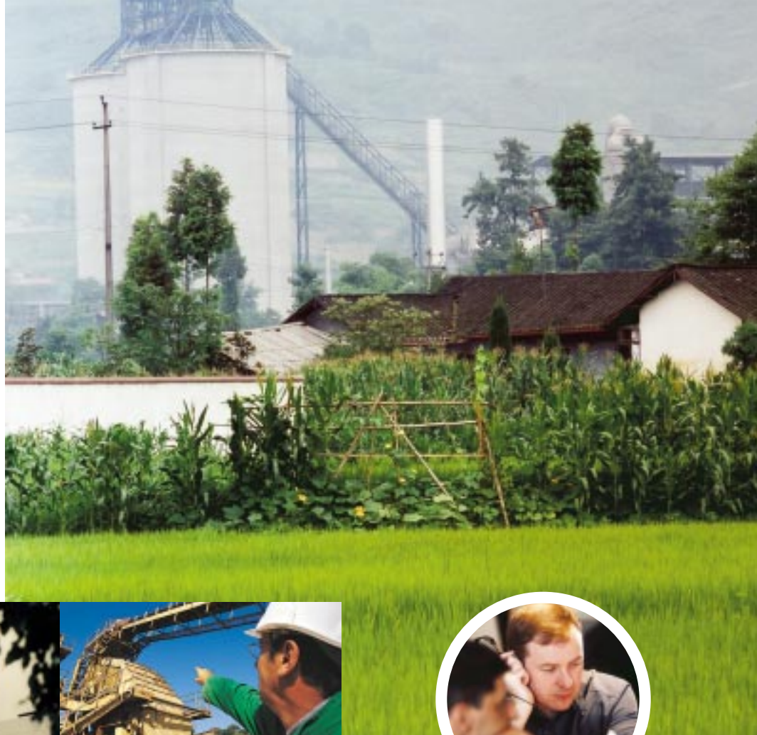
China / Cement. The Dujiangyan cement plant.
