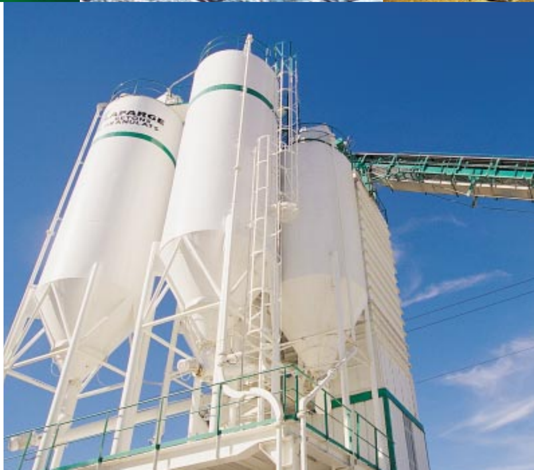
France / The Pierrelatte concrete plant.
