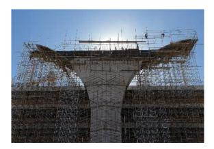
Duracem cement is used to mix concrete that is particularly strong, hard and durable. As it is also self-leveling and hardens on its own, this considerably reduces the work on the thin prestressed concrete structures.
