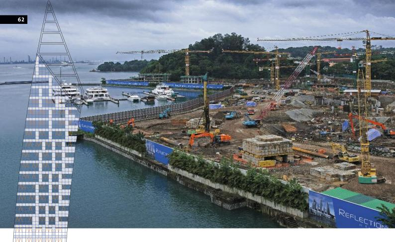
site, and made available from two new metering and mixing plants with a total production capacity of 240 cubic meters an hour. The plant also runs on weekends and holidays whenever required. The Holcim truck fleet transports some 300 to 500 cubic meters of concrete to the building site every day. "The developer, the investor and the architect expect top-notch quality, reliable service and 24-hour delivery capability", says Jitendra Pragji Desai. "We can guarantee all of that."
